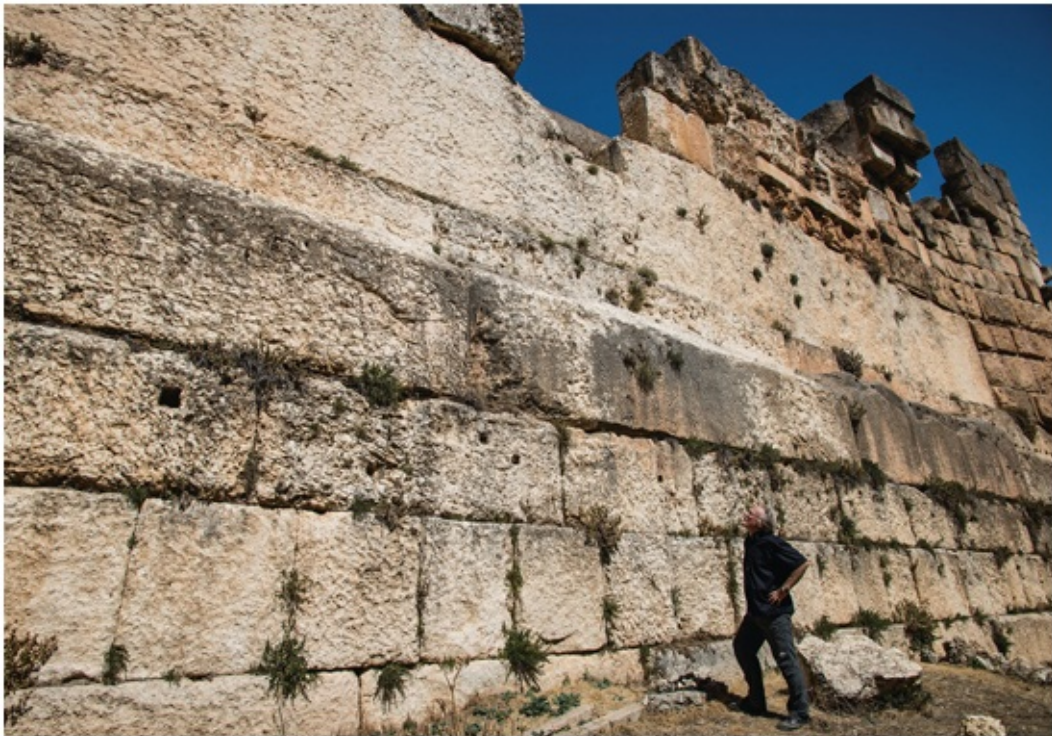
40. The author's right foot is placed in front of the fragment of a Roman column drum used as a block in the foundations beneath the Trilithon.
