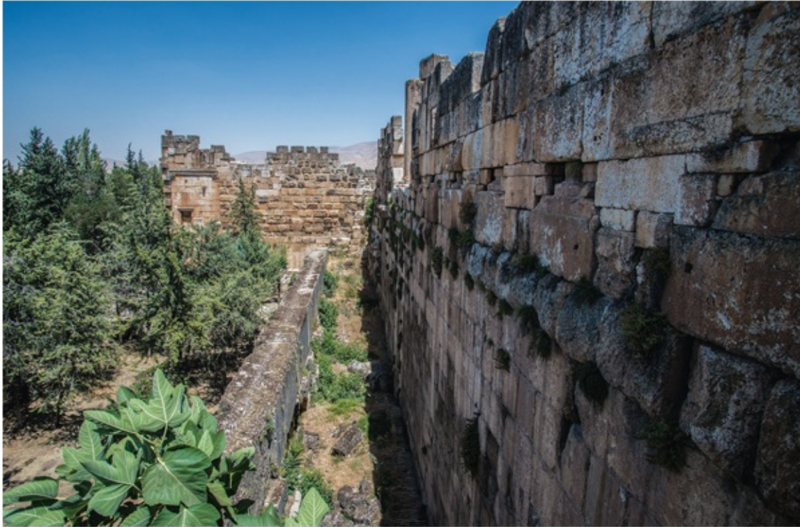
44. Northern arm of the U-shaped megalithic wall surrounding the platform of the Temple of Jupiter. Note the smaller size of the blocks with which the platform itself (right side of picture) is built.
