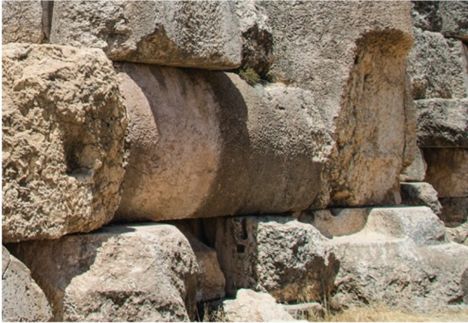
43. Close-up of the recycled column drum in the Arab fortification wall. Note the drum is perfectly flattened at top and bottom exactly like the column drum in the foundations beneath the Trilithon. The argument that the Arabs lacked the technical expertise to cut and fit blocks so precisely therefore makes no sense.
