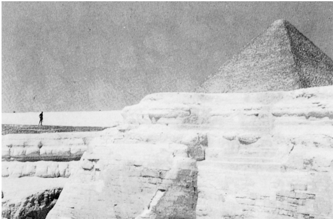
71 The rear of the pit or trench out of which the body of the Sphinx was carved again shows the characteristic vertical fissures and scalloped coves of precipitation-induced weathering. The rump of the Sphinx, also shown, has been partially covered in repair blocks in modern times.
