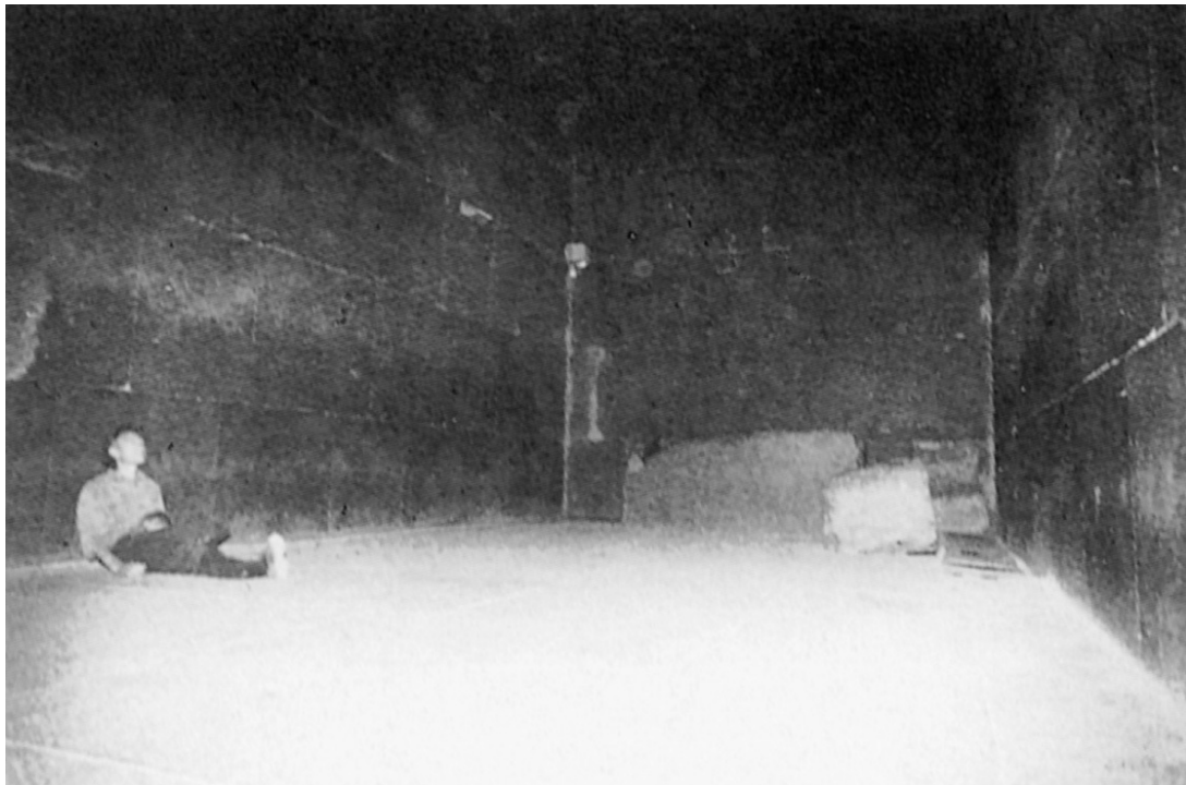
44 The author in the King's Chamber in the heart of the Great Pyramid. The walls are composed of 100 separate blocks weighing around 70 tons each, and the ceiling is spanned by 9 further blocks each weighing 50 tons. The engineering logistics involved in creating such a chamber at a height of 150 feet above the ground are stupefying.
