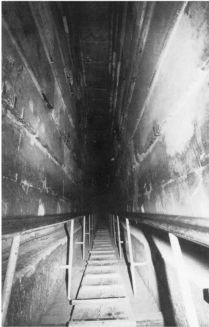
46 The Grand Gallery. Are we looking down? Or up? Measuring 153 feet in length, and 28 feet high, this awe-inspiring corbel vault has an angle of slope of 26^\circ and represents a near-impossible engineering and architectural feat.
