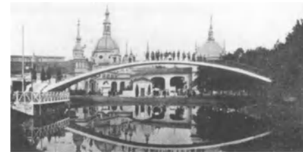
Bremen, bridge by G. Wayss, 1890, 40 m
