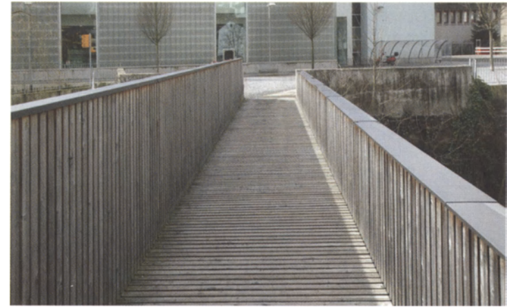
View towards the shopping centre
