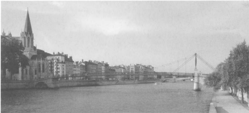
Passerelle Saint Georges, 1852, 87.5 m free span
