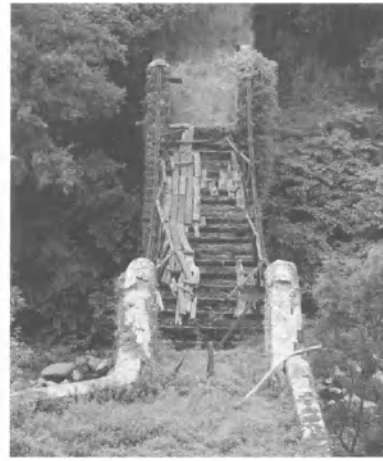
Suspension bridge over the Cance in Annonay, 1822
