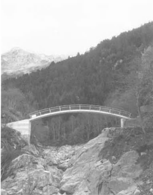
Passerelle SOJ, Val Soj in Ticino CH, 2006
