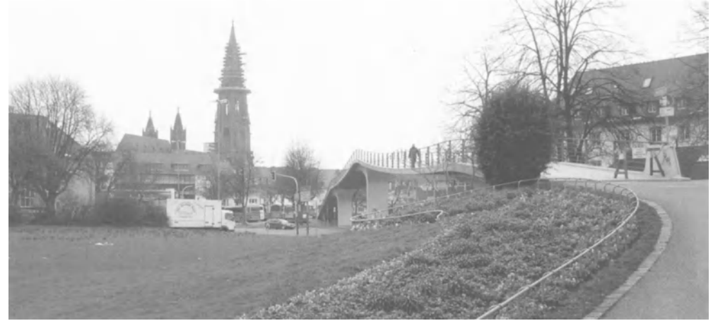
Stress Ribbon Bridge in Freiburg, Germany, 1970
