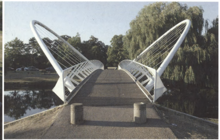
Arches – 1888 vertical, 1997 inclined
