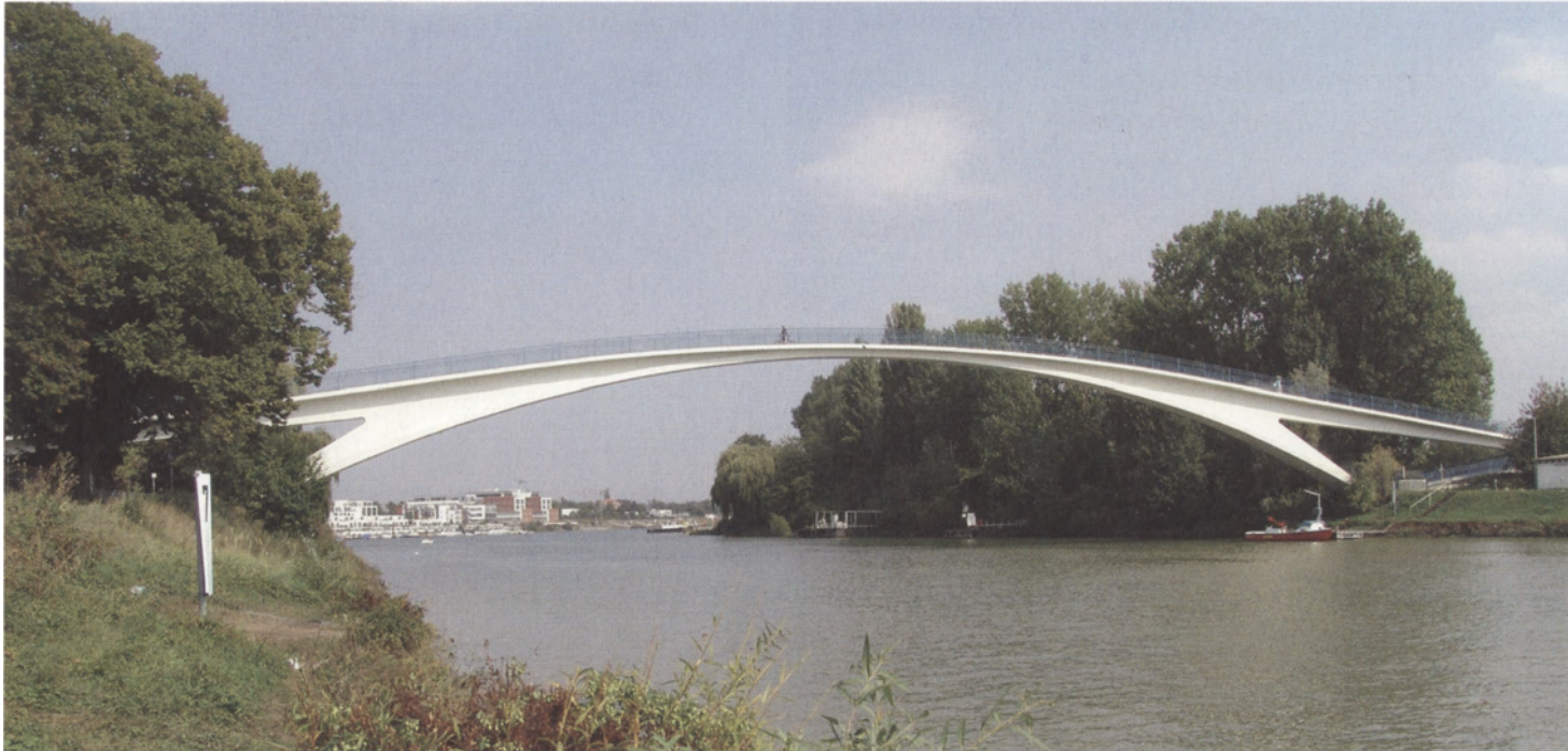
Schiersteiner Footbridge, Wiesbaden, Germany, 1961
