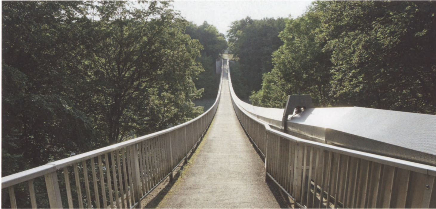
Stress Ribbon Bridge in Geneva, Lignon-Loex, Switzerland, 1971
