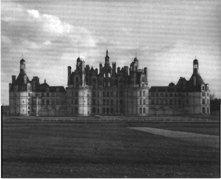
Plate 4 North-west façade of the Château at Chambord, France. Photo © Lonchamp Arch.Phot.Paris/SPADEM, © C.N.M.H.S./SPADEM
