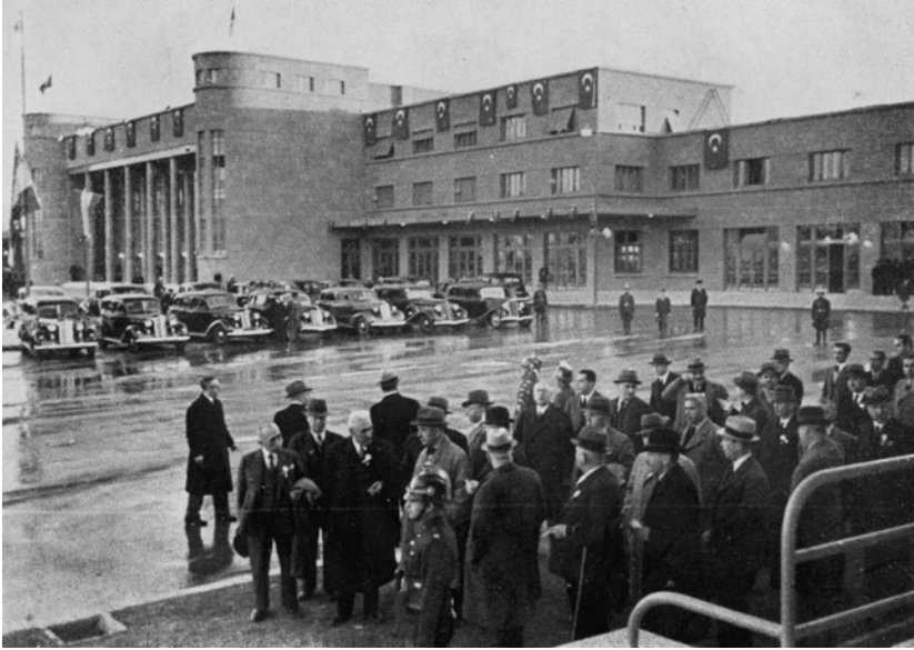
Fig. 16.6 Opening of the Ankara railway station (1937) designed by Şekip Akalın [Fotoğraflarla Yeni Ankara Garı, official photo album, author's collection]
