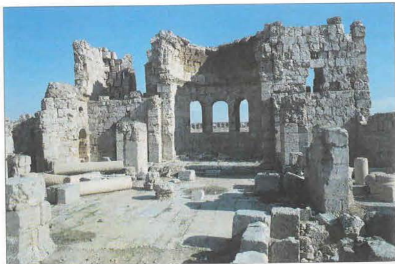
Right: the early 6th-century church of St Sergius and Bacchus at Rasafah, an important late Roman garrison town in Syria. The west end of the church was formed by a pair of towers; at the east end, the semi-circular apse was covered by a half dome.
