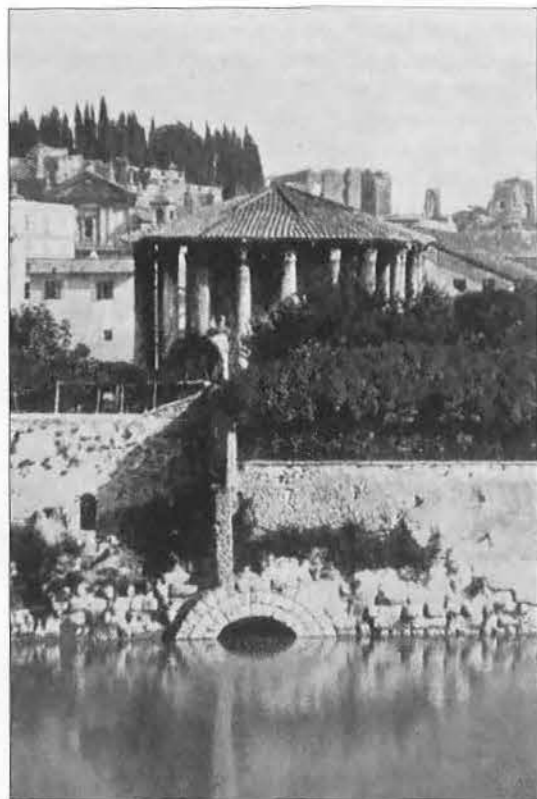
Above: the heart of Republican Rome, seen from the River Tiber. Opening into the river is the mouth of the Cloaca Maxima, the great sewer which drained the valleys between the hills of Rome, making possible the laying out of the Forum. Originally built by the Etruscans, it was substantially repaired during the reign of Augustus (27 BC–AD 14). Above it is the round temple of Hercules Victor, built in the late 2nd century BC.
