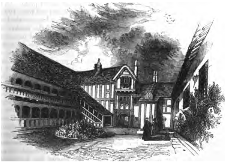
Leicester's Hospital, Warwick.
