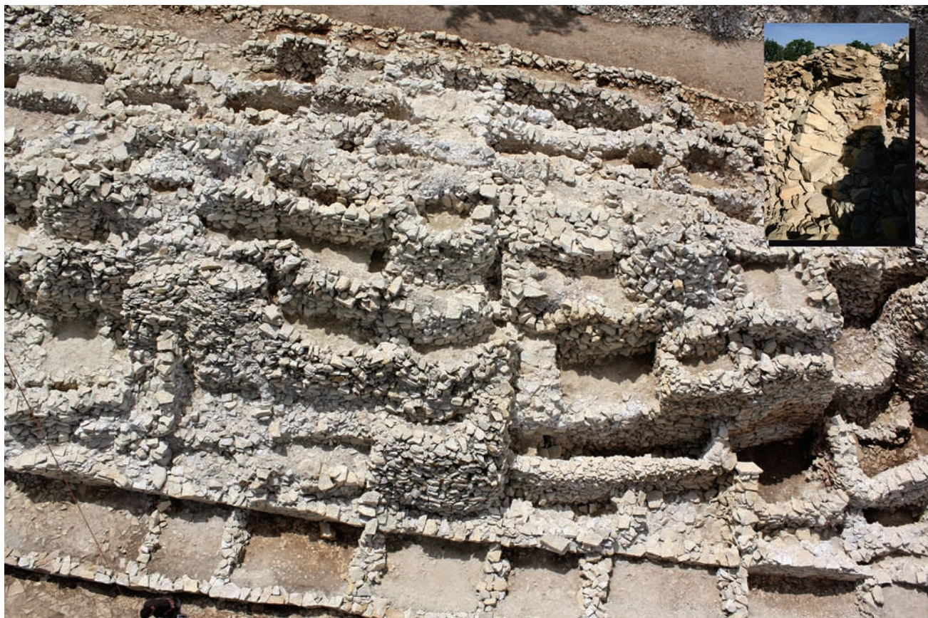
Fig. 2.5: Elevation of the cairn: tiering of relieving arches on the northern face at the eastern end of Péré tumulus C at Prissé-la-Charrière, Deux-Sevres, France (L. Laporte)
