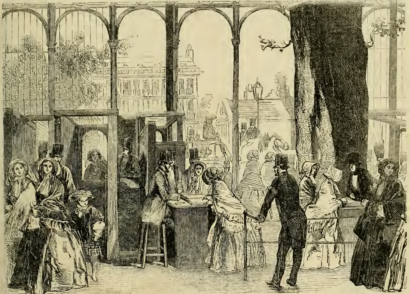
THE SOUTH ENTRANCE, AS SEEN FROM THE INSIDE.
