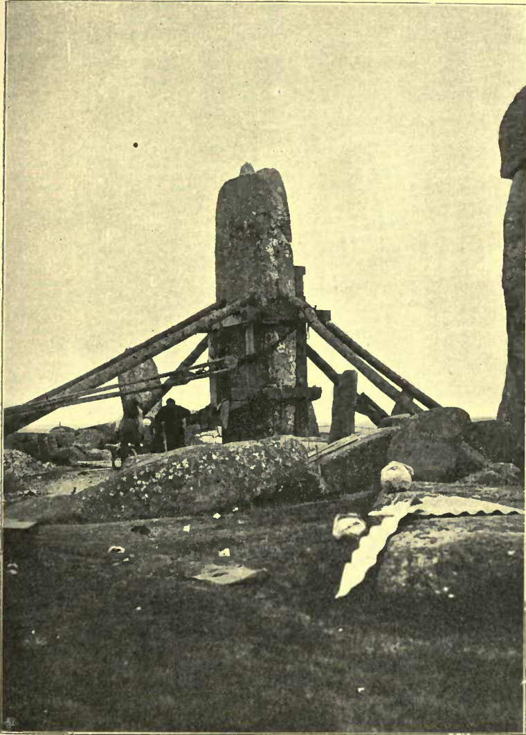
FIG. 22.—The leaning stone upright before the struts were removed.
