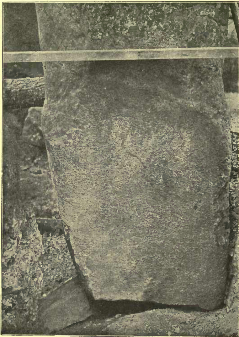
FIG. 8.—The original tooling of the stone protected from the action of the weather.
