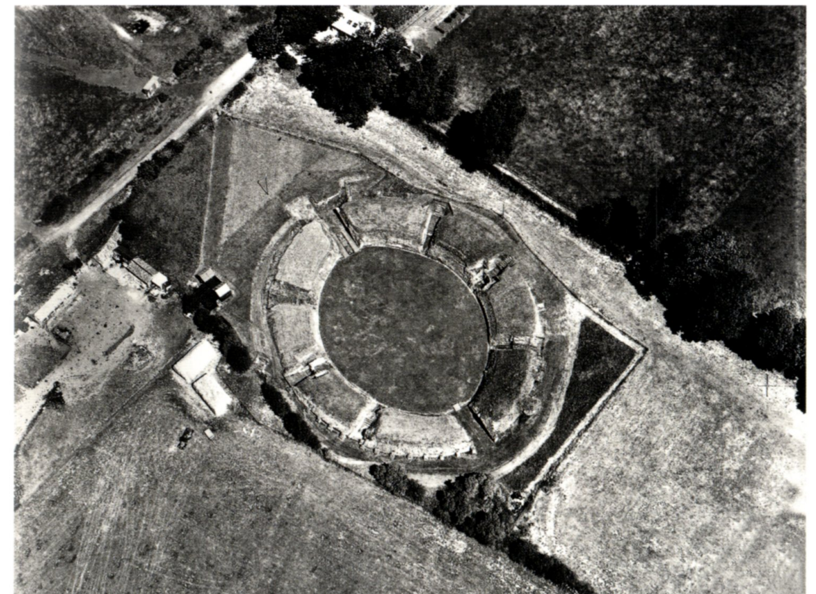
120. Caerleon (Monmouthshire). The legionary amphitheatre at Caerleon, built c. 90, for II Augusta . The arena was created by hollowing out the ground, and seating was built out of stone-revetted earthen banks.
