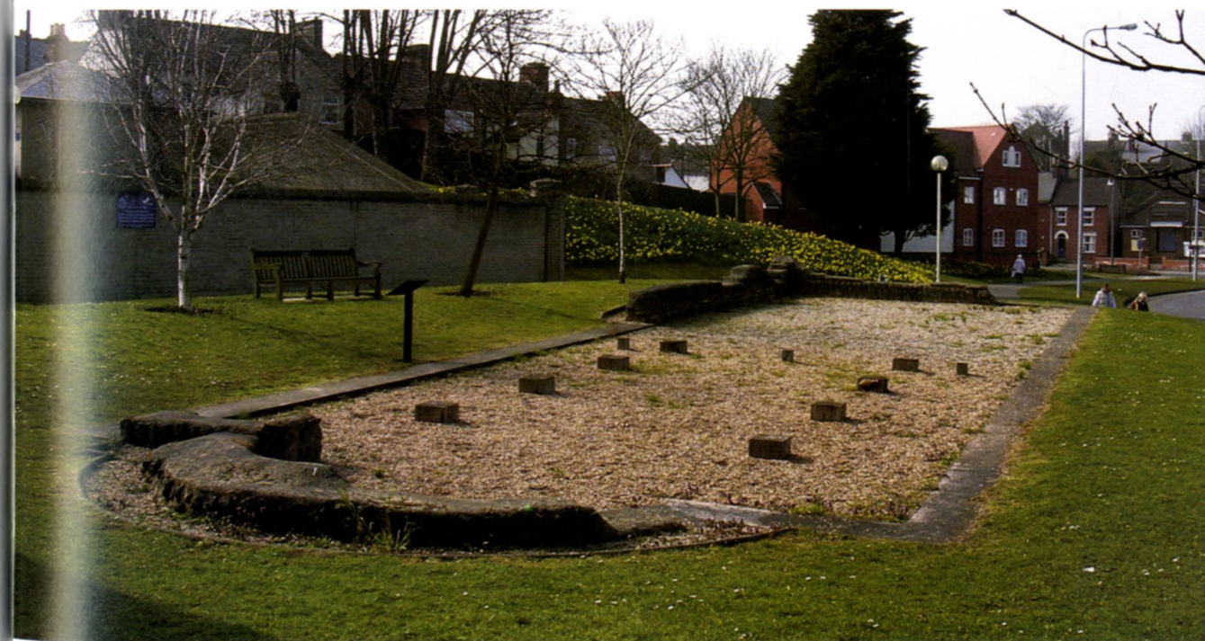
237. Colchester (Essex). This 'church' has been identified as such because of the ground plan and clustering of late Roman east-west graves around it. Built about 320–40, with the apse added c. 380.
