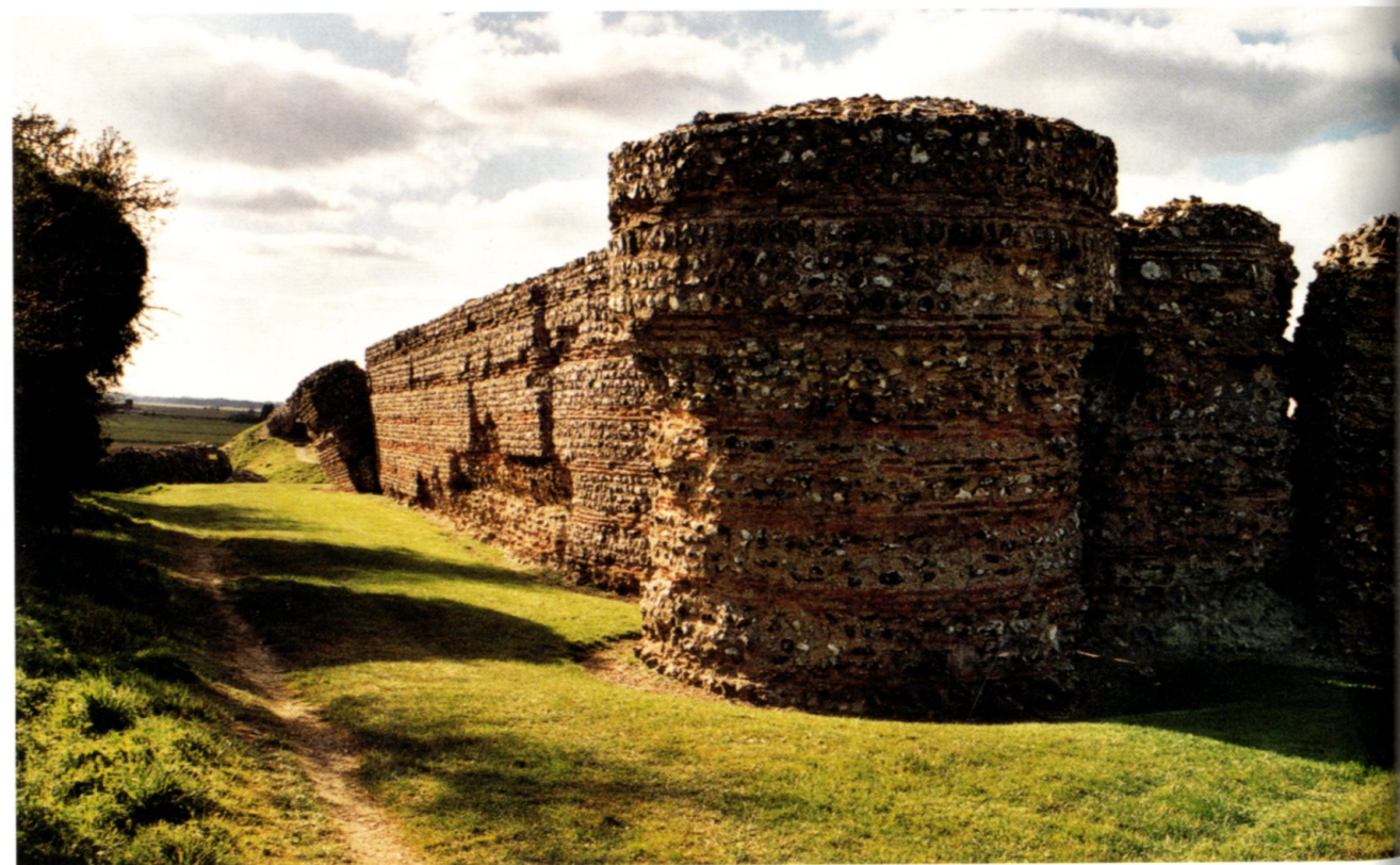
121, 122. Burgh Castle (Suffolk). The shore fort defences at Garriannum . Built c. 275, the fort appears to show a transitional design. The bastions were added after the walls had been partly built, and are only bonded to the upper courses.
