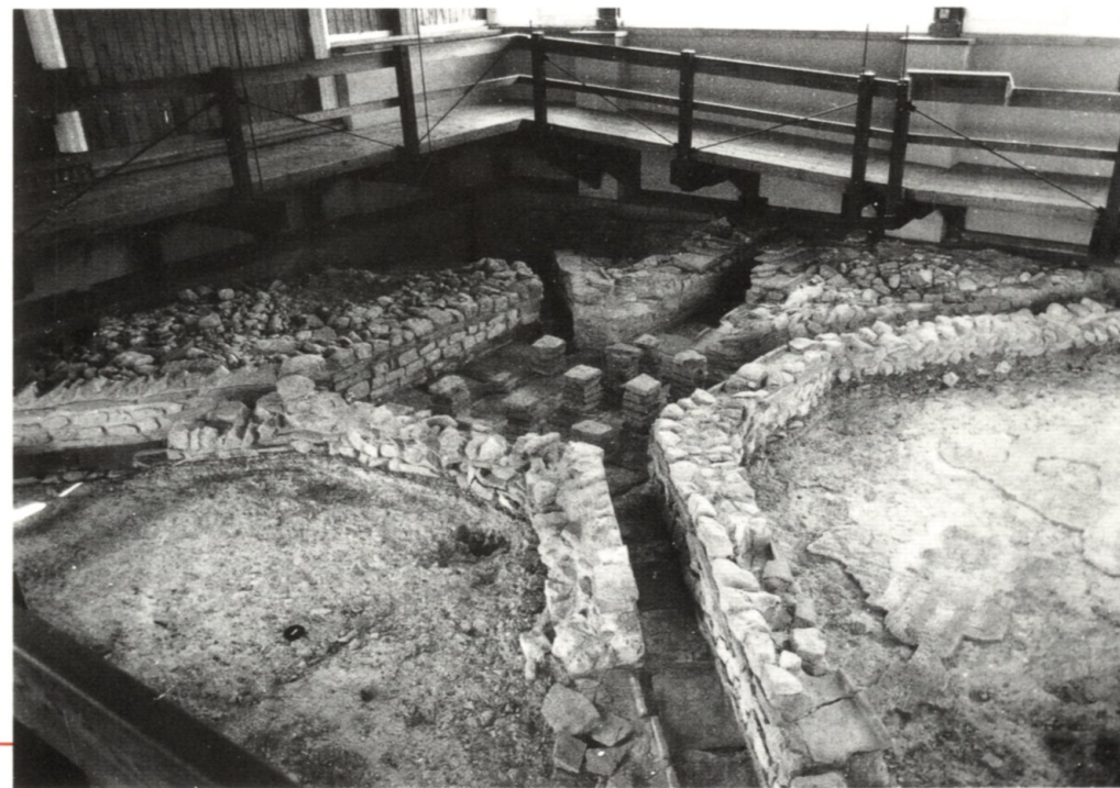
198. Hypocaust system. Second-century underfloor heating at Fishbourne Palace, installed during a series of modifications.
