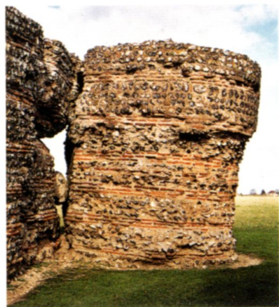
121, 122. Burgh Castle (Suffolk). The shore fort defences at Garriannum . Built c. 275, the fort appears to show a transitional design. The bastions were added after the walls had been partly built, and are only bonded to the upper courses.
