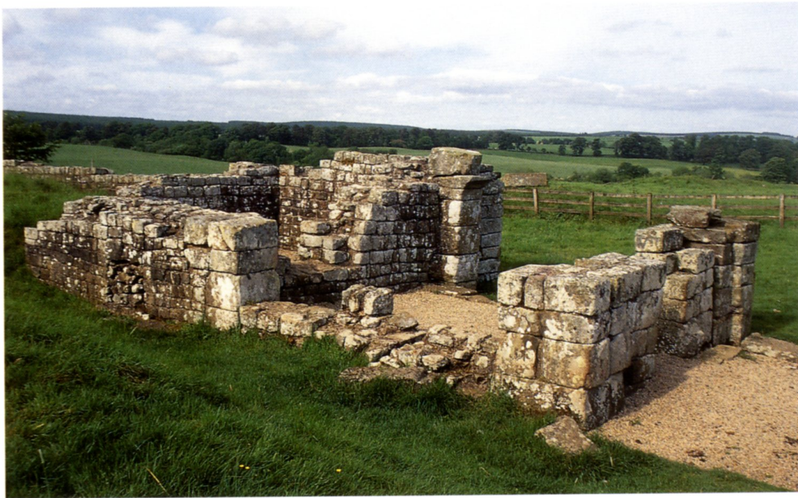
114. Birdoswald (Cumbria). The double-portalled east entrance to the fort at Banna is the best-preserved fort gate in Britain, still standing to the height of its arch springers.
