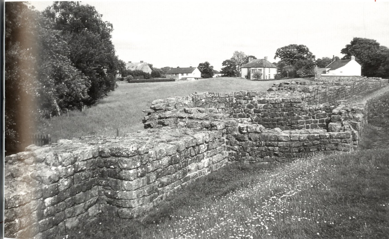
48. Right. Willowford (Cumbria). Turret 48a was built in expectation of the Broad Wall, but the change of plan to the Narrow Wall resulted in the offset.
