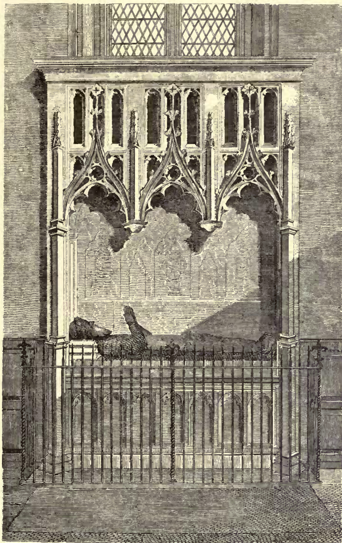
GOWER'S MONUMENT, ST. MARY OVERIES
