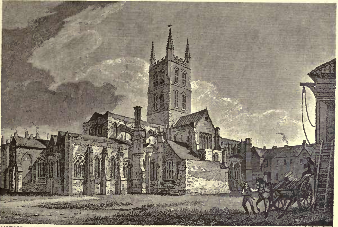
NORTH EAST VIEW OF ST SAVIOUR'S CHURCH.
