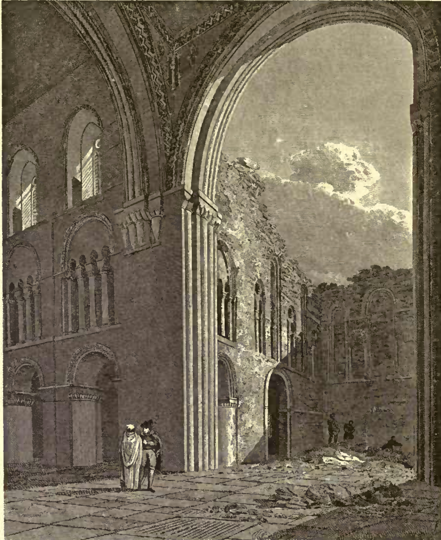
PART OF With the REMAINS of the SOUTH TRANSEPT IN WEST
