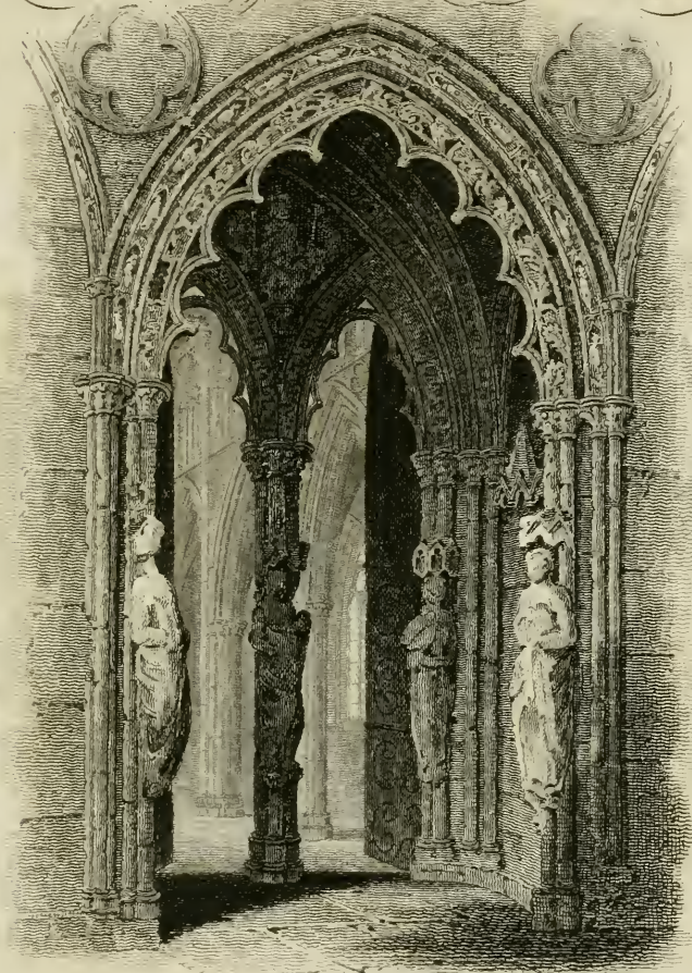
West-door Lichfield Cathedral.
