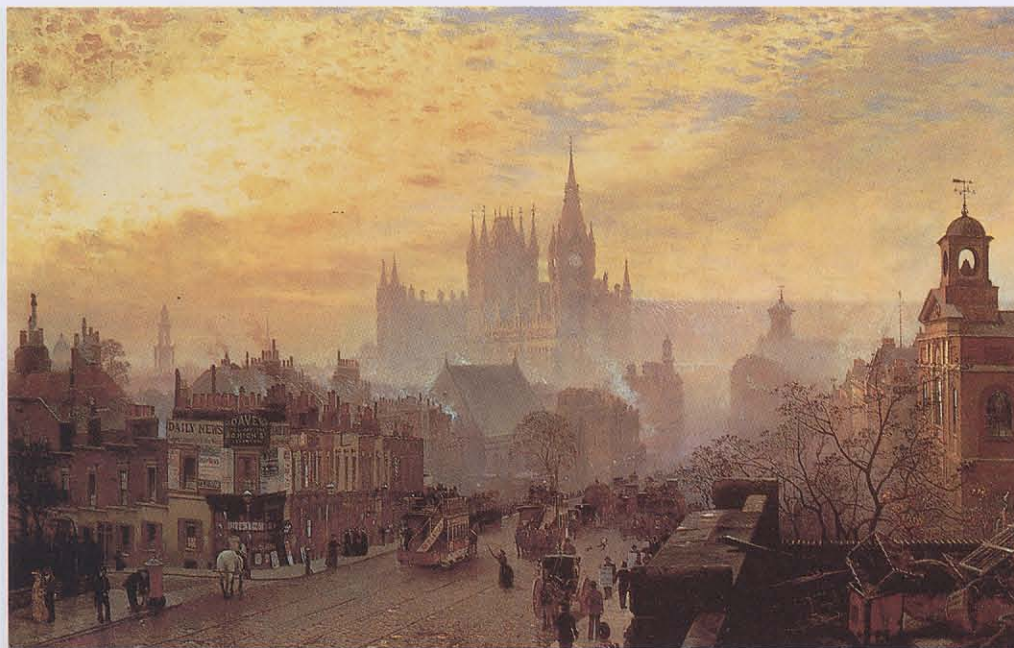
Much of London still looks as it did in the closing years of the nineteenth century. "St Pancras Hotel and Station from Pentonville Road: Sunset" by John O'Connor (1884) shows St Pancras as it was meant to be seen, a temple to Victorian values towering above the surrounding houses. St Pancras, built by George Gilbert Scott, is one of London's finest "Gothic revival" buildings.
