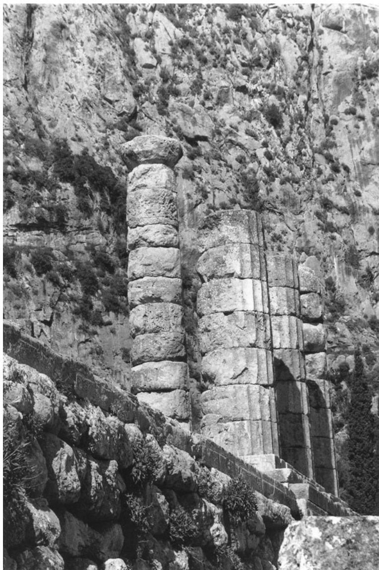
FIGURE 4.23. View of re-erected columns of the Apollo Temple. The column drums are chipped along both bottom and top edges, evidence of the twisting and shaking they underwent from the earthquakes that overthrew them. The columns stand on a tall podium, which adapts the steep hillside to the support of the building. Three steps (stylobate) elevate the columns above the platform.
