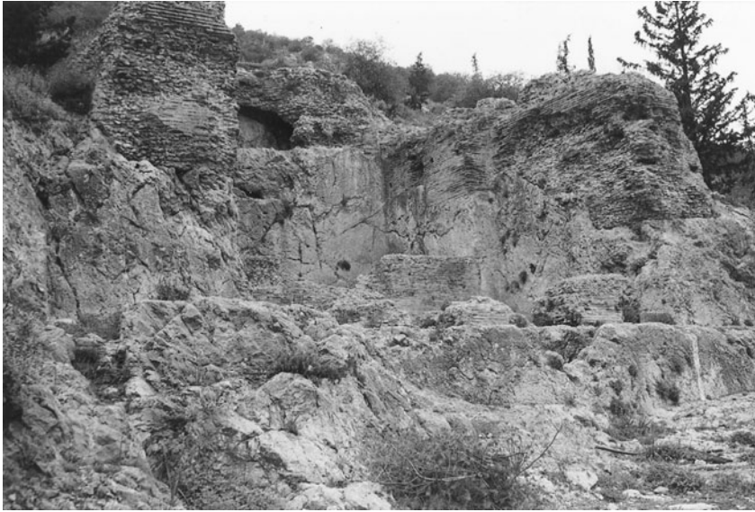
FIGURE 4.5. ( continued ) Photo of Kritērion fountain. Water once emerged from between the two kinds of rock visible here; the fountain appears to have been developed around an original spring. In addition, the second-century C.E. aqueduct was led to feed the upper part of the fountain, where massive brickwork extends the fountain's walls upward. (Photo by Crouch)
