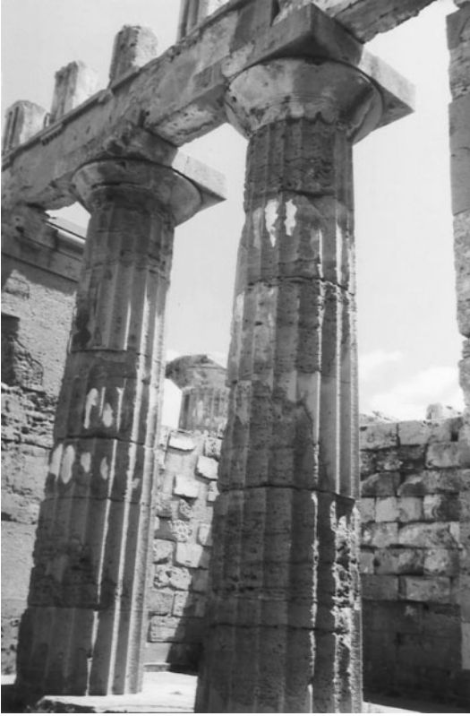
FIGURE 1.1. Columns partially covered with stucco, at Selinus. (Photo by Crouch)
