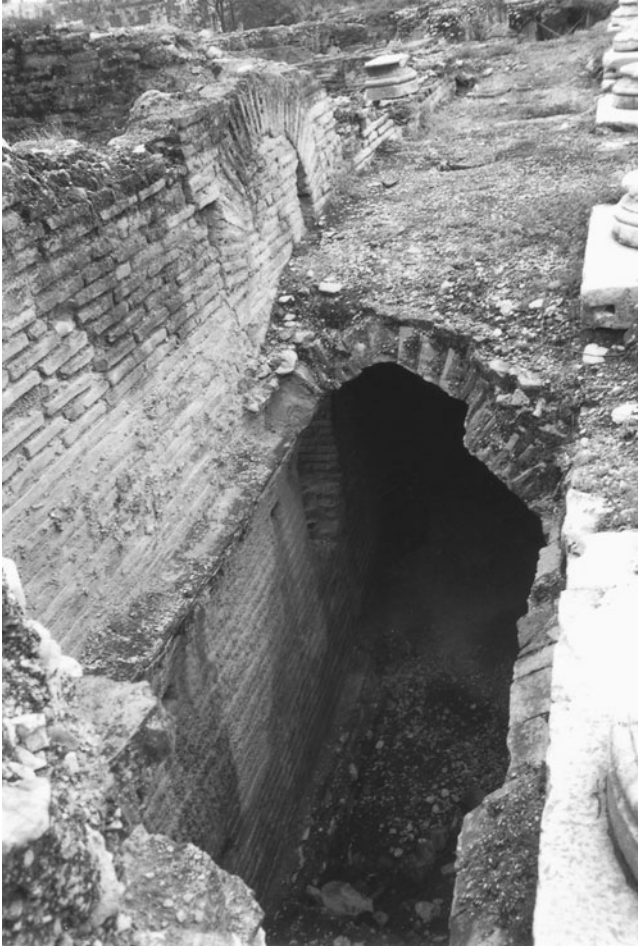
FIGURE 4.7. Photo of the drain tunnel from the Roman bath at Argos, similar to the set of three large drains in the agora. The tunnel is tall enough for a medium-size adult to walk upright in. Drains of this time, made with brick vaults, are assumed to be Roman. (Photo by Crouch)
