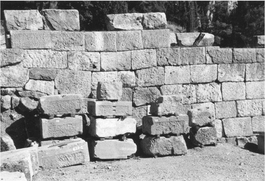
FIGURE 4.20. Deformation of a wall, produced by earth movements, in Apollo sanctuary area. (Photo by Crouch)
