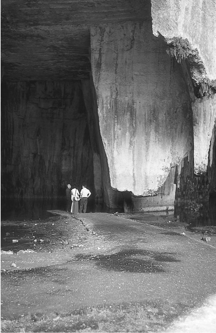
FIGURE 3.28. Quarry (latomia) in Syracuse. Cut into karstified limestone, the quarry collects water draining from the plateau. The stone of the piers splits off, forming reverse stair steps. This photo was taken in 1977. Earthquakes have caused ceilings and piers to fall in, so tourists are no longer allowed to enter the area. (Photo by Crouch)
