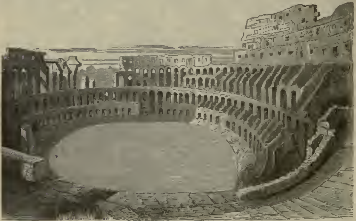
FLAVIAN AMPHITHEATRE IN ITS PRESENT CONDITION (1879)—INTERIOR.
