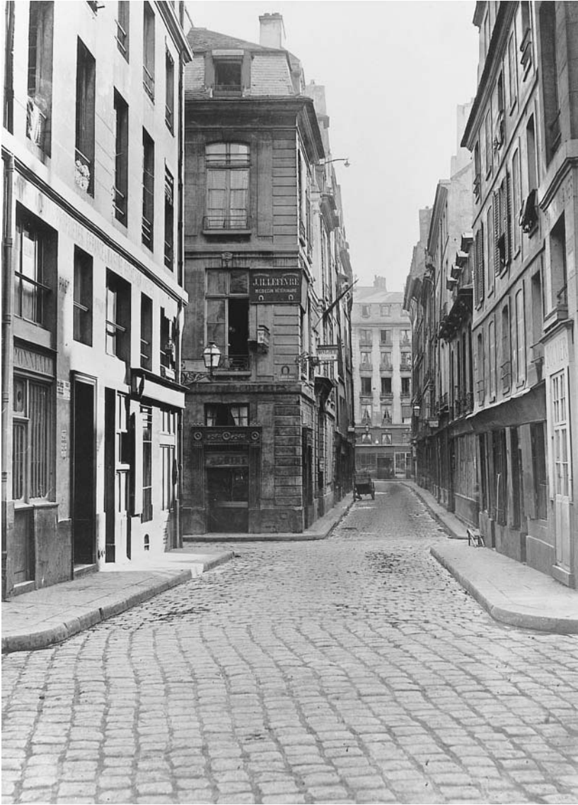
Figure 29. Rue Sauval. The older section of seventeenth-century houses in the background contrasts with the wider eighteenth-century street in the foreground, part of the speculative housing development around the new grain market. The chemist and fermier général Antoine Lavoisier grew up in the rue Sauval and lived most of his life in the quarter. Original photo by Charles Marville, ca. 1864. Bibliothèque historique de la ville de Paris, photo Jean-Christophe Doerr.
