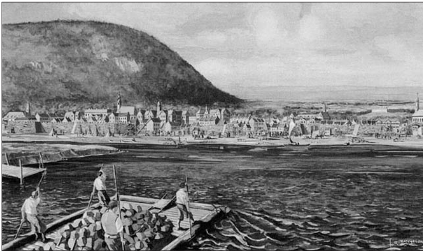
Building the walls at Montréal, 1717–44. In the foreground, a large raft brings stones to be used to face the wall under construction from the west (left). The small citadel is at the eastern end (right). Mount Royal is visible in the background. (Painting by L.R. Batchelor c.1933; National Archives of Canada, C1540)
