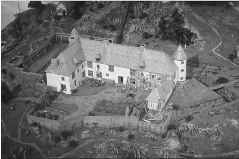
The second “Habitation” was built in 1624–26 and replaced the first one built in 1608. Situated at the foot of Cape Diamond, it was larger and featured two medieval-looking stone turrets at the corners of a large stone building enclosed by a wooden wall. At the time, Québec was primarily a fortified trading post. (Model at the Centre d’Interprétation de la Place Royale, Québec; Author’s photograph)
