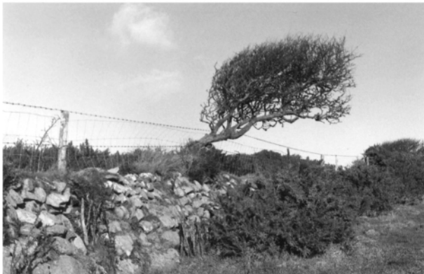
Figure 3.13 Tresyssylt, West Wales, field walls showing a diversity of sequence. Upper: gorse, thorn bushes and fencing. Middle: large grounders, smaller stones and turf bank with gorse. Lower: stone bank, turf bank, thorn bush and fencing.
