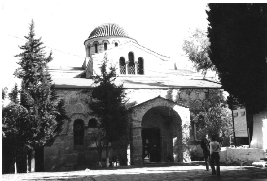
Figure 7.6 Byzantine Church of Panagia Scripou at Orchomenos, Boeotia; inscriptions were incorporated in the wider context of the re-use of spolia from the ancient acropolis and theatre. Upper: detail of column segments, tile and stone. Lower: general view of the west end.
