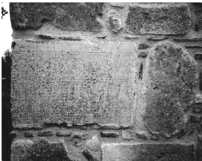
Figure 7.7 Panagia Scripou, Orchomenos; inscriptions on the outside of the church. Upper: use of tile and small stone. Lower: use of tile, carefully prepared blocks, and irregular stone.
