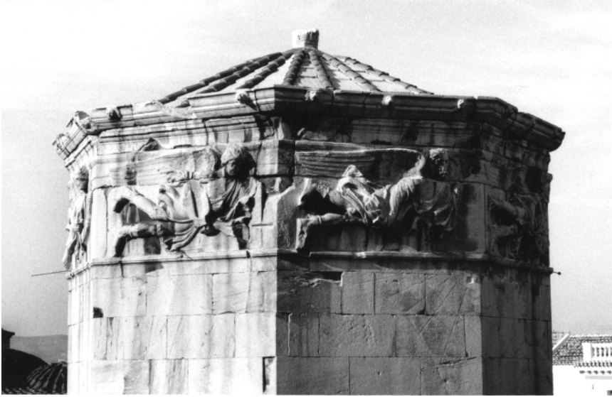
Figure 5.1 Tower of the Winds or Temple of Aiolos, Roman agora, Athens, an octagonal tower with depictions of the winds on its eight faces. It was used as a sun clock in the manner of a sundial, and some of the inscribed marker lines can be seen on the nearest face.
