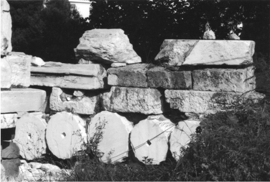
Figure 2.1 The re-use of antiquity. Late Roman wall in the Athens agora, built around AD 280, showing the re-use of ancient building materials, including column segments.
