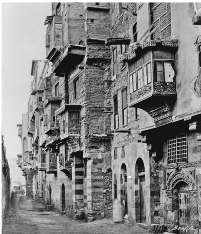
Taken in the 1880s, this photo shows a street in the Ibn Tulun quarter of Cairo. Traditionally, the houses in Cairo were several stories high and were made of mud brick with stone facades on the ground floor. The wooden window projections on the upper floors, known as mashrabiyya , allowed the women of the house to watch the street action without being seen. (Photograph by Maison Bonfils, courtesy of the University of Pennsylvania Museum, Philadelphia)
