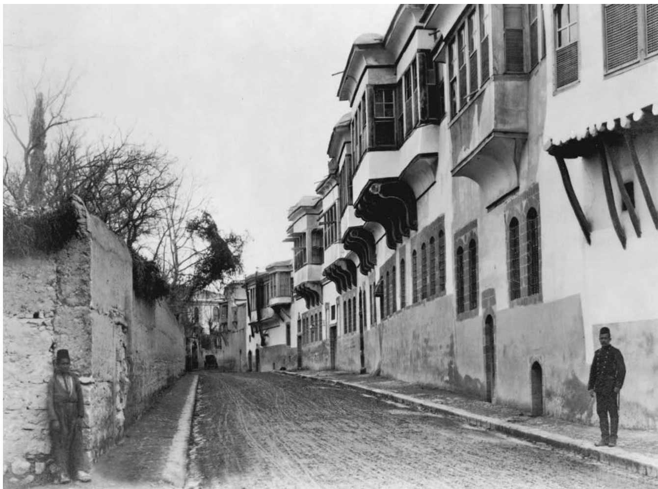
After the riot of 1860, wealthy Damascenes moved out of their old-style courtyard houses in the walled city to the suburban quarter of Salihyya where houses in the late Ottoman style were constructed along paved streets. This photo dates from the 1880s. (Photograph by Maison Bonfils, courtesy of the University of Pennsylvania Museum, Philadelphia)
