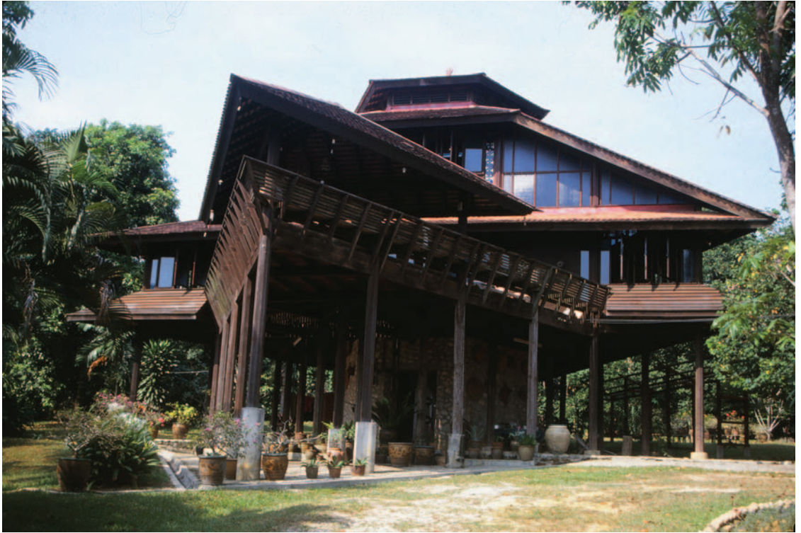
The Salinger House Kuala Lumpur-based architect Jimmy C.S. Lim has created a contemporary translation of the traditional Malaysian house, for Rudin Salinger and his wife, on a site that was once part of a rubber plantation, south of the old capital city. He had introduced exciting new elements into the historical model, making it fresh and yet still comfortably familiar. Source: James Steele
