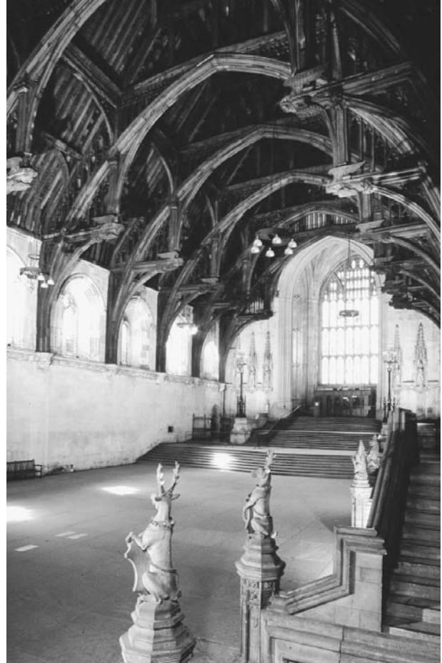
Interior of Westminster Hall showing hammer-beam wooden roof structure and stalls, London, England, 14th century. ADAM WOOLFITT/CORBIS.
