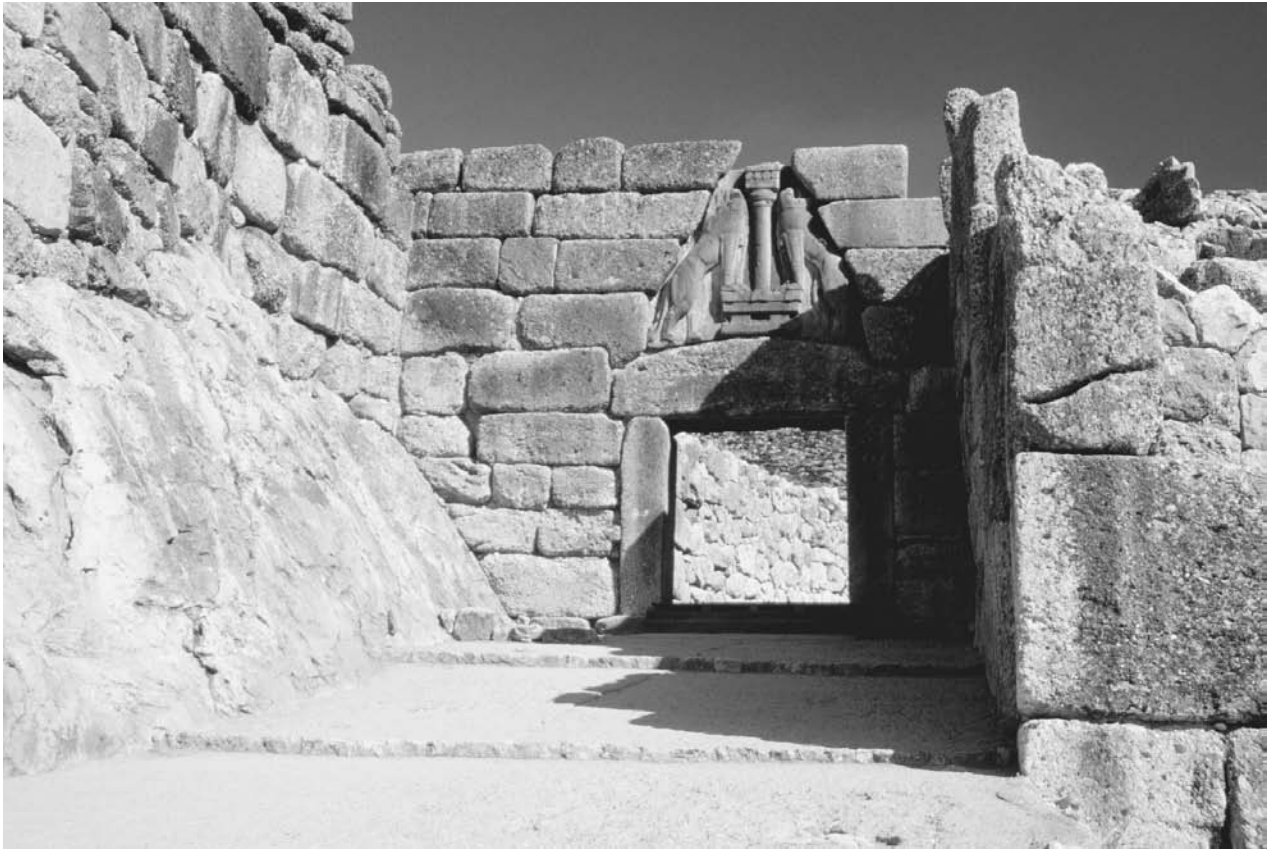
The Lion Gate at Mycenae, Greece, so-called from the sculpture on the limestone slab above the lintel block, showing two lions with their feet resting on an altar. © CHRIS HELLIER/CORBIS.
