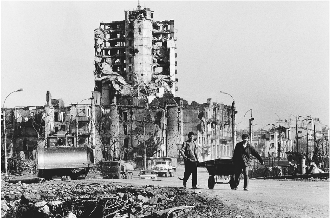
Grozny, Chechnya, after its destruction by Soviet bombing, April 1995. Here, two of the capital's survivors begin the grim task of rebuilding. [TEUN VOETEN]
