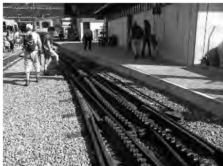
Fig. 62. Cogwheel railway in Switzerland
