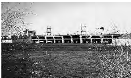
Fig. 151. Hydroelectric power station at the Dniepr river
