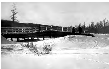
Fig. 146. Hazard of aufeis: Destruction of a bridge by the river aufeis at a tributary of Amur river
