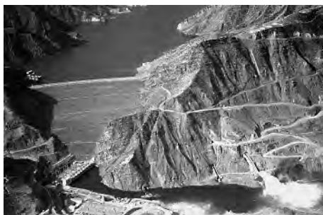
Fig. 356. Water spill (right down) at the Nurek hydroelectric power station, Tajikistan
