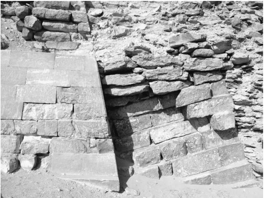
Step Pyramid of Saqqara. The blocks composing this early pyramid were angled inward, rather than leveled, to prevent its collapse. Photo courtesy of Pat Remler.
