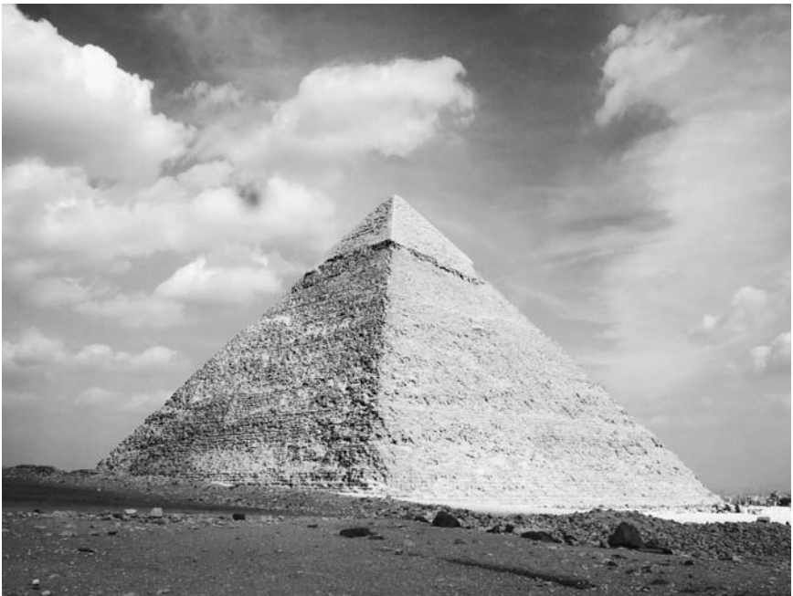
The original outer limestone casing is still visible at the top of Chephren's pyramid. Photo courtesy of Pat Remler.
