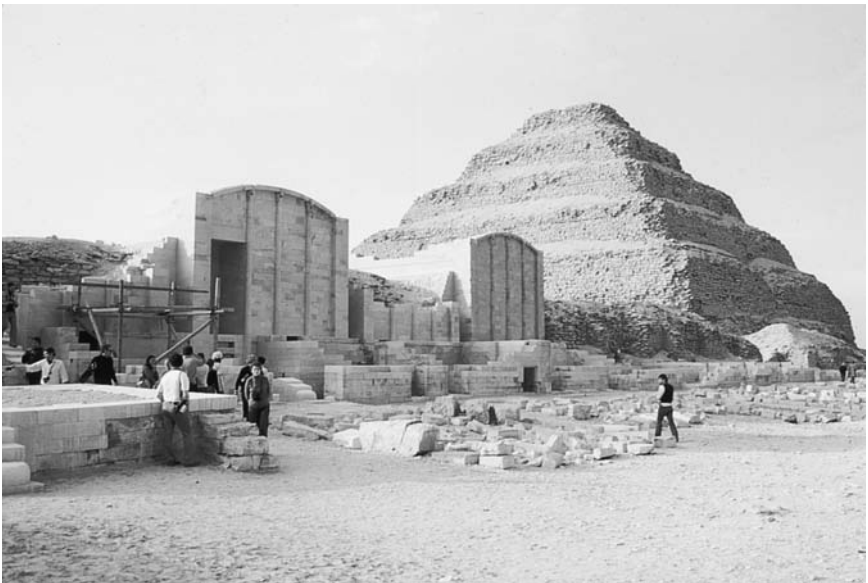
The Step Pyramid at Saqqara, the oldest large building in stone. Two dummy temples in solid stone appear in the foreground. Photo courtesy of Pat Remler.
