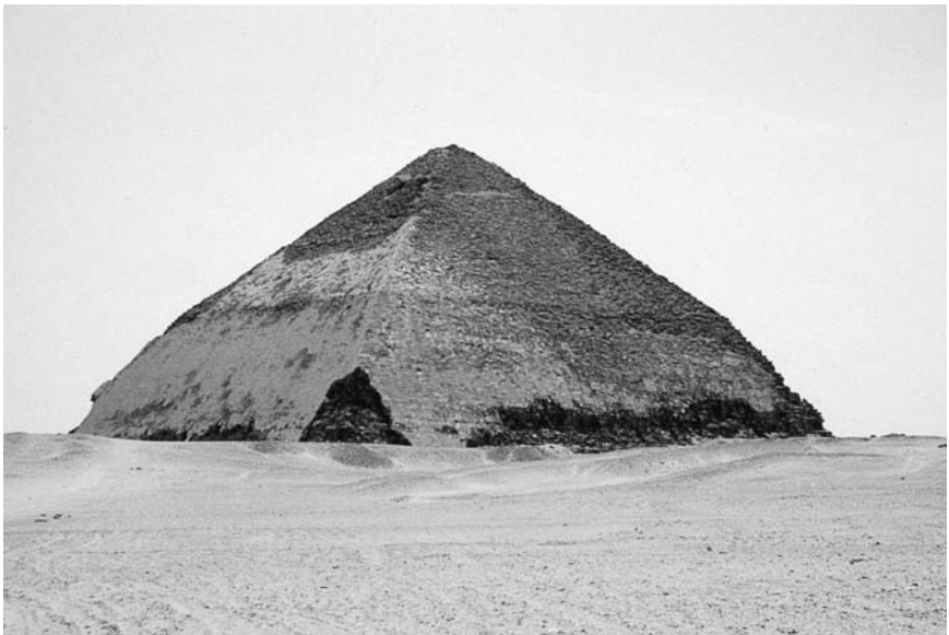
Silhouetted against the sky, the change in angle of the Bent Pyramid is clearly visible. Photo courtesy of Pat Remler.
