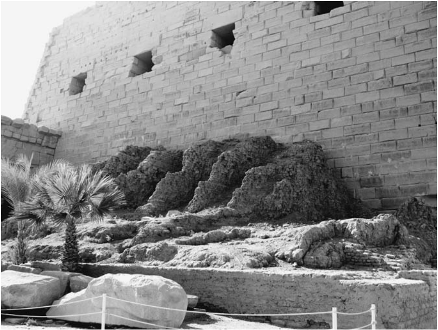
The eroded remains of a mud brick ramp used to haul stones to the top of one of the pylons (gateways) to Karnak Temple. Photo courtesy of Pat Remler.
