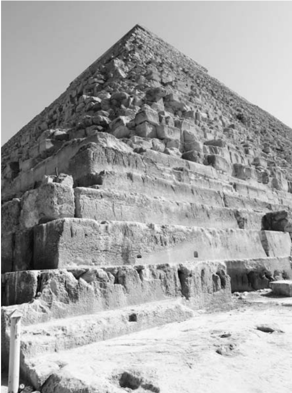
Chephren's Pyramid. Today this pyramid looks "stepped" because the smooth white outer casing stones used to produce a smooth face were removed and used for building later structures. Photo courtesy of Pat Remler.
