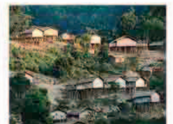
▲ This stilt village in Bangladesh is built to resist the regular flooding. Pressure on land, even in rural areas, forces many people to live in marginal areas.
