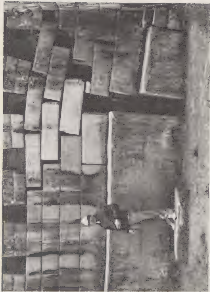
A rectangular-construction wall, split during a massive earthquake. Note that the irregularly-shaped megalithic walls would survive better. The largest block, behind explorer Richard Kieninger, weighs approx. 150 tons.
