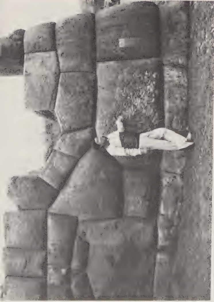
Detail of a megalithic wall at Sacsayhuaman. Each oddly-shaped block fits perfectly with the others, making the wall earthquake-resistant. The larger blocks in this photo all weigh well over ten tons.
