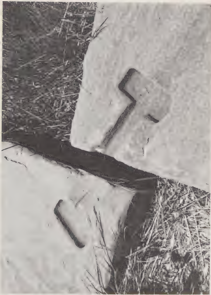
A keystone cut in the blocks at Puma Punku. An unusual and sophisticated method for fastening megalithic blocks together, a similar cut can be found at Ollantaytambo.
