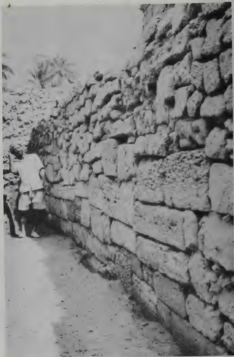
At least four thousand years old (and probably older) this wall at Qala'at al-Bahrain still survives to an appreciable height. From Looking for Dilmun .
