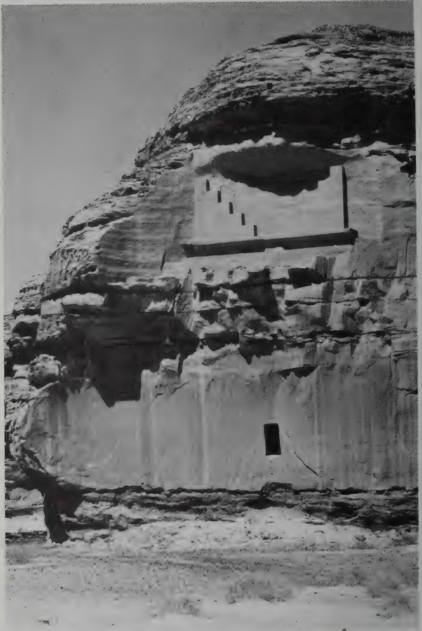
Another cut stone building at Mada'in Salih. This was obviously part of a greater structure which interlocked with other walls now gone. Vanished in a cataclysmic upheaval?
