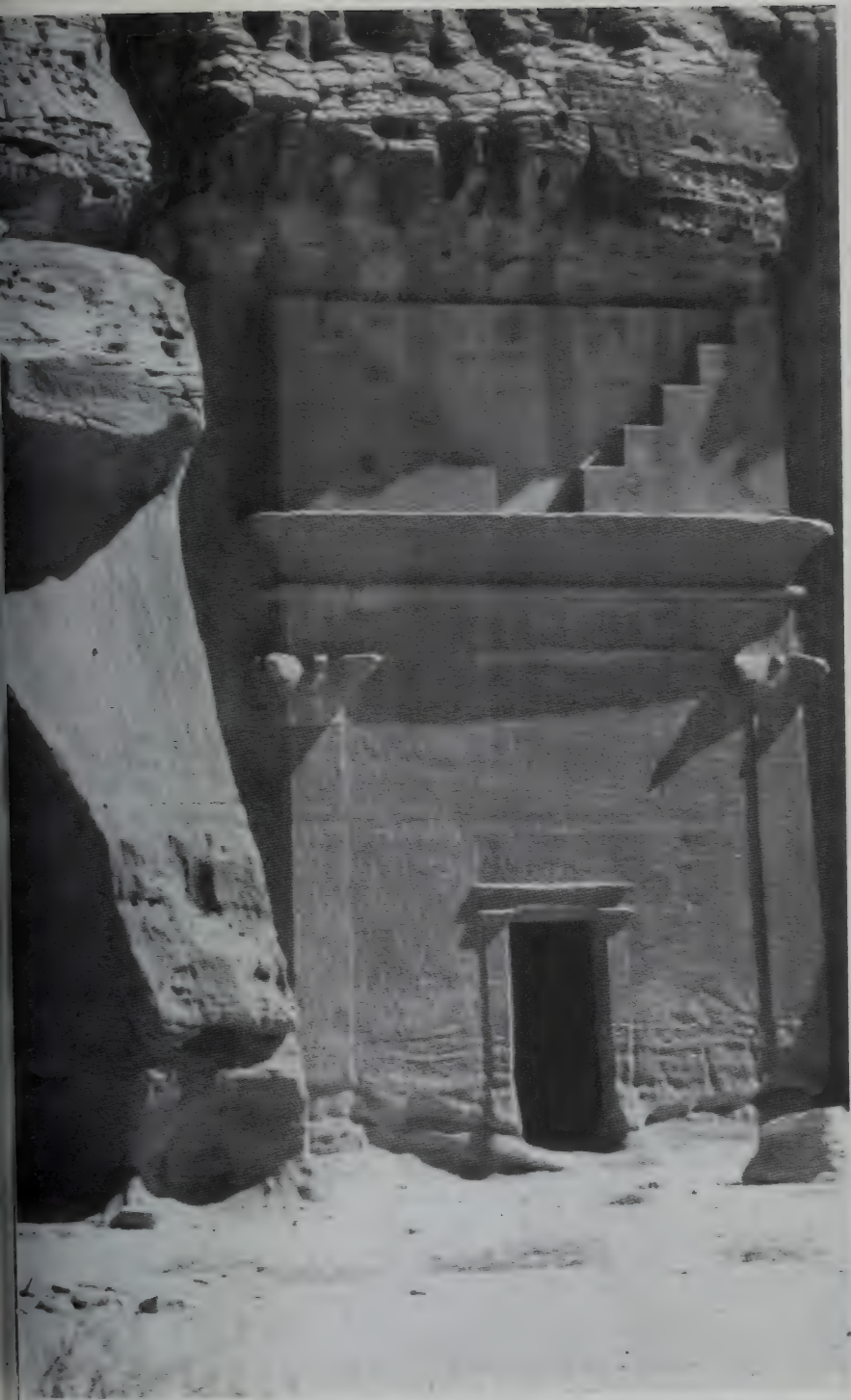
One of the facades at Mada'in Salih, Saudi Arabia, cut into the rock face. Like Petra in Jordan, it is attributed to the Nabateans. Note the severe weathering, as if by water, on the lower part.
