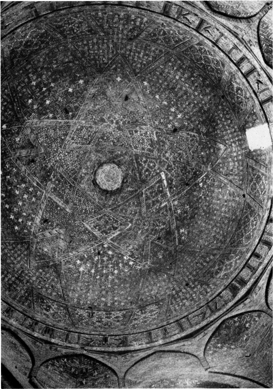
5 Isfahān, north dome, from inside.
