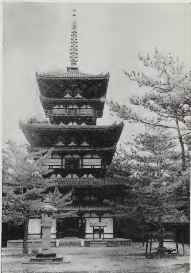
The three-storied Tōtō (Eastern Pagoda) of the Yakushiji Temple, Nara, appears to be a six-storied structure, because of the mokoshi (intermediate projections) protruding from each floor.
