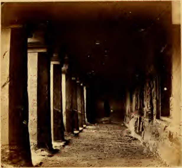
INTERIOR OF VERANDAH, CAVE No. 4.—AJUNTA.
