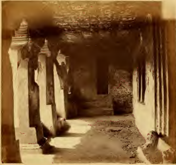
VERANDAH OF CAVE No. 11.—AJUNTA.
