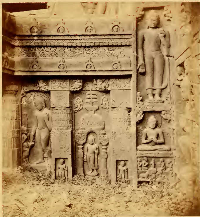
LOWER PART OF FACADE OF CHAITYA No. 19.—AJUNTA.
