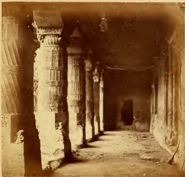
INTERIOR OF VERANDAH, CAVE No. 1.—AJUNTA.
