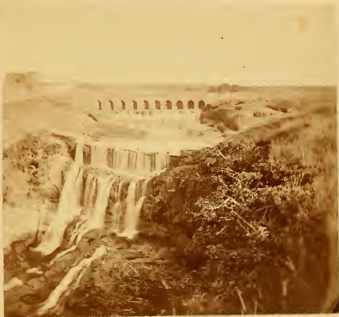
BRIDGE AND TOWN OF AJUNTA.
