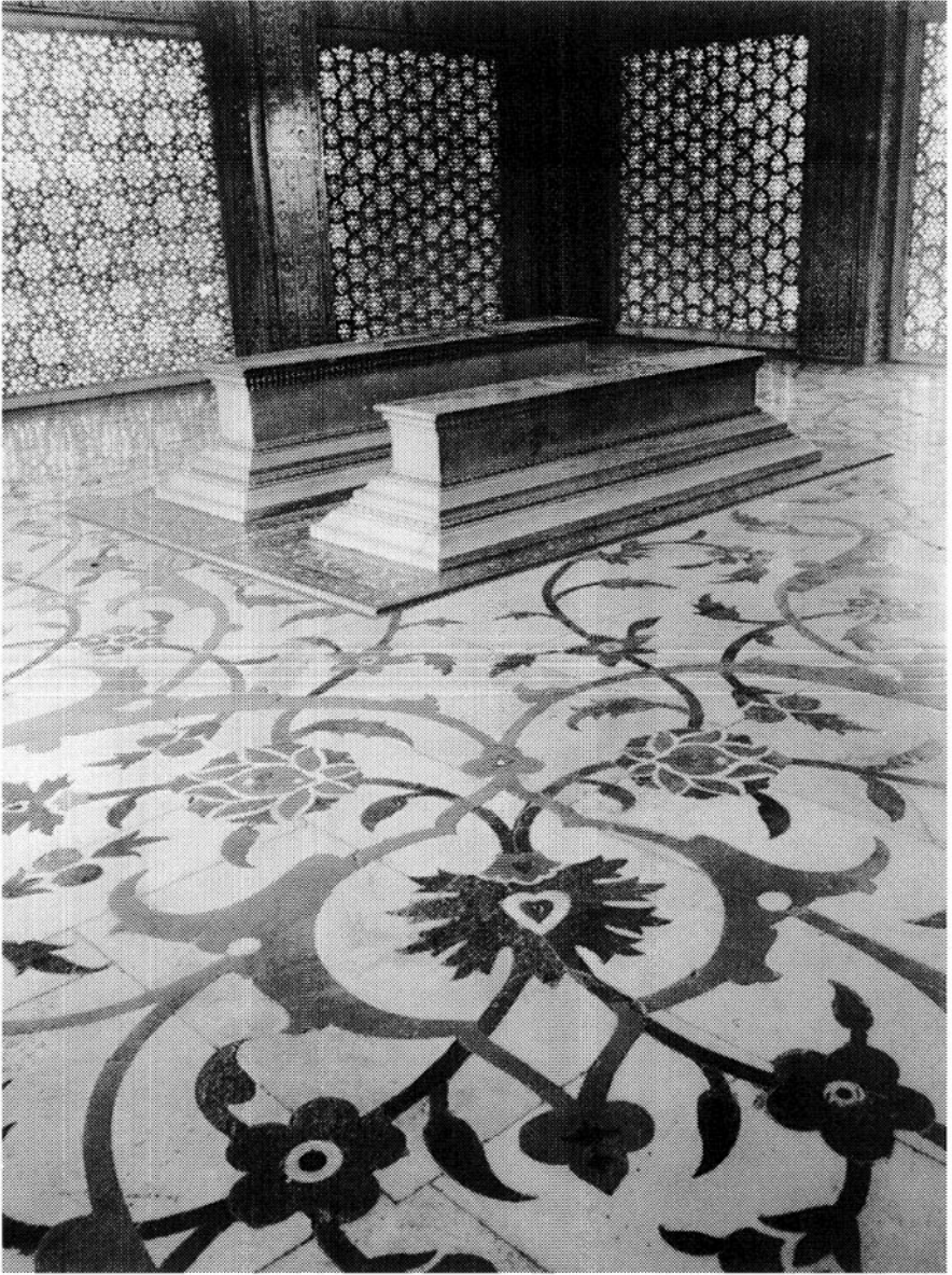
FIGURE 9-4. Floor and lattice patterns around cenotaphs of Itimaduddaula and Asmat Begam in upper pavilion of Itimaduddaula's tomb, Agra. Courtesy of the Archaeological Survey of India, New Delhi.
