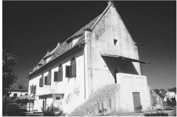
A Dutch trading building in the former colony of Sulawesi, Indonesia. (JEREMY HORNER/CORBIS)
