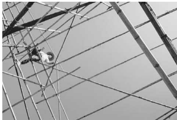
Bamboo has many uses in Asia. Here, a man climbs on a bamboo construction scaffolding in Hong Kong. (TRAVEL INK/CORBIS)
