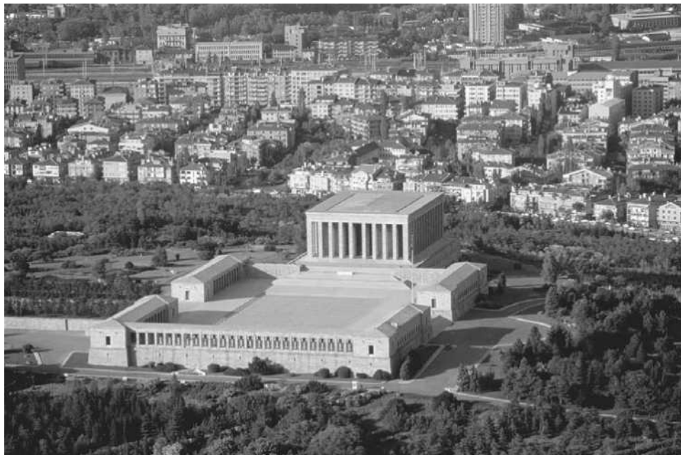
An aerial view of the mausoleum of Kemal Ataturk, the founder of the Republic of Turkey, in Ankara. (YANN ARTHUS-BERTRAND/CORBIS)
