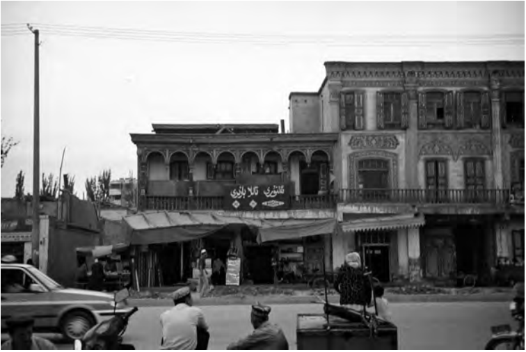
Older, run-down buildings in a Uighur section of Kashgar.
