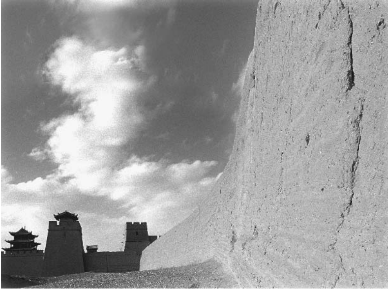
The fortress at the western end of the Great Wall, whose rammed-earth construction is clearly visible
