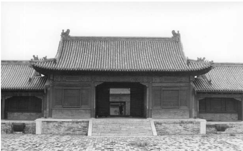
Inner part of the Forbidden City, Beijing. The Qing left this Ming palace unchanged
