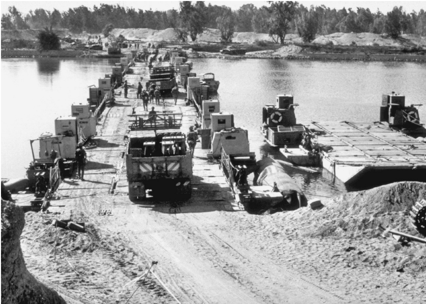
Temporary bridge across the Suez Canal allowing Israeli troops to cross to the western side during the Yom Kippur War (Courtesy Embassy of Israel, Washington, D.C.)
