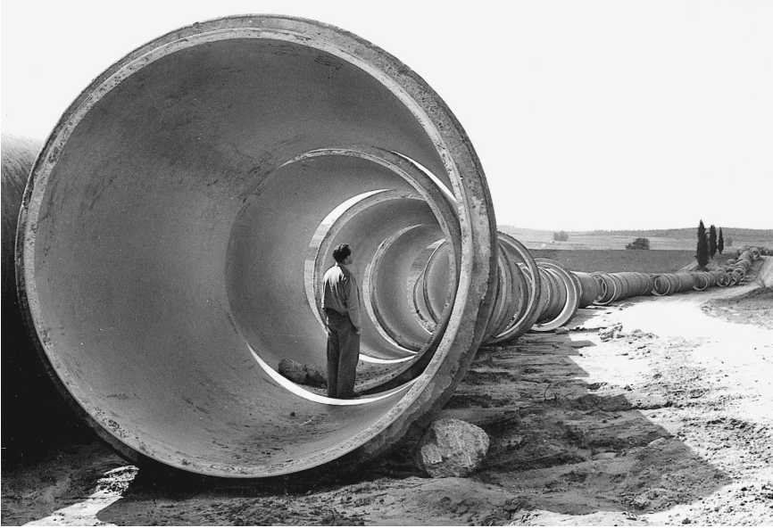
Water pipes for Israel's National Water Carrier (Courtesy Embassy of Israel, Washington, D.C.)
