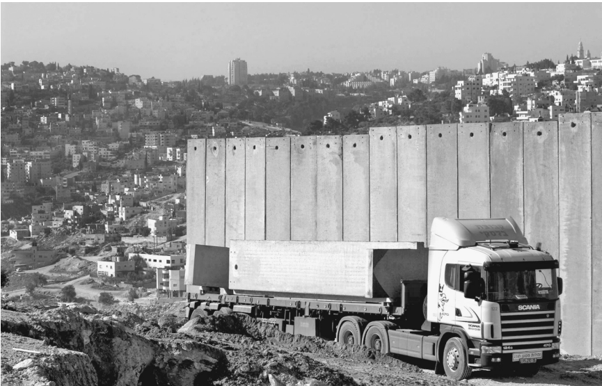
The security fence separating Israel from the Palestinians in the West Bank; the photos illustrate the two main forms of construction—fence (top) and concrete barrier (below)—used depending on the terrain and population locations. (Israel National Photo Collection)
