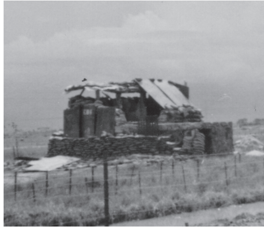
Bunker 051, outside Tan Son Nhut Air Base, which was overrun and destroyed by the enemy during the Tet Offensive. Three men were killed, including a close boyhood friend of the editor. (Courtesy Salvatore Raffa)
