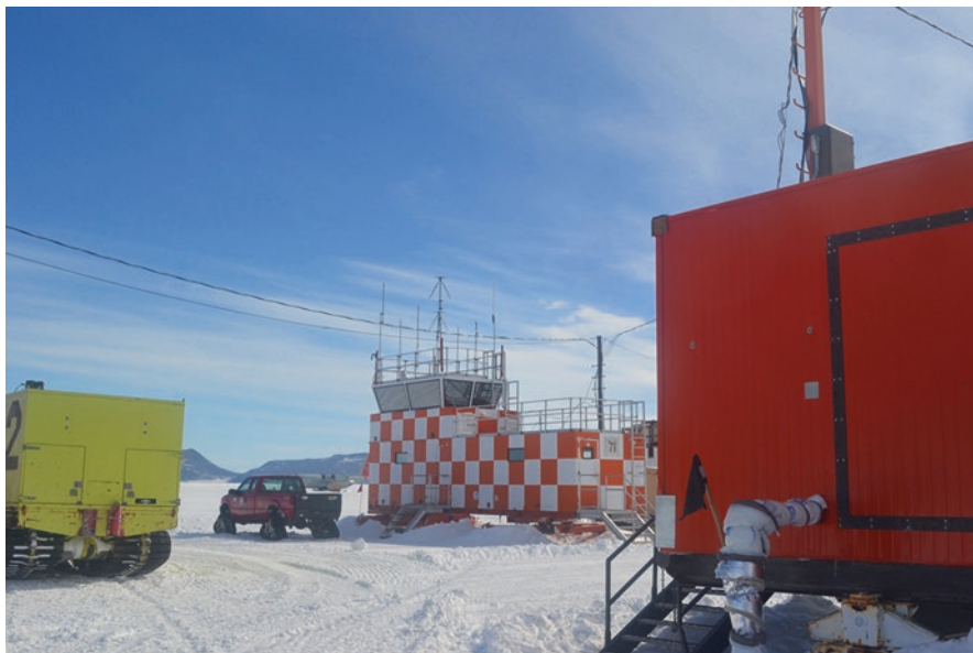
Fig. 1.9. The buildings of Williams Airfield rest on skids for easy movement (Photo by the authors)
