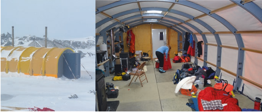
Fig. 6.8. Two views of the Rack Tent. Notice the blue “airlock” entrance. The interior shot was taken at 10:30 pm, lit only by natural light filtering through the skylights (Photo by the authors)
