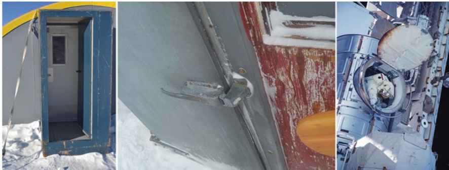
Fig. 4.5. (Left) A blue, double-doored “air lock” at the front of a rigid tent near the Lower Erebus Hut on Mt. Erebus; (Center) A typical “freezer-style” door handle in Antarctica; (Right) An astronaut exiting the Quest airlock on the International Space Station (Left, center photos by the authors; right photo courtesy NASA/JSC)
