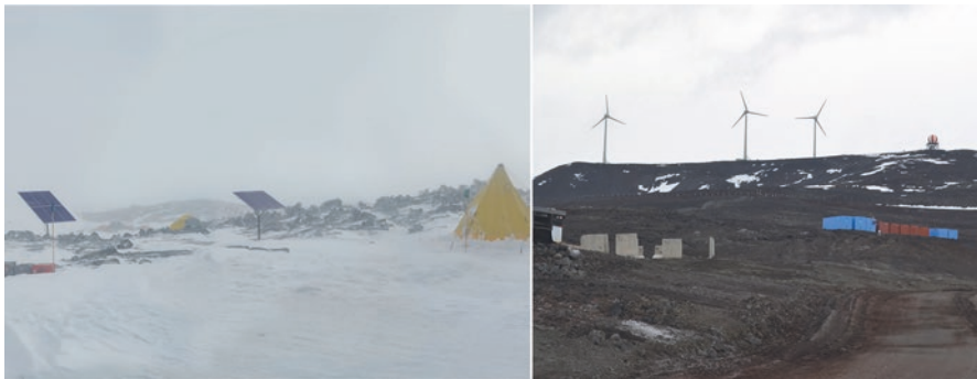
Fig. 4.8. Two sources of power in Antarctica: ( Left ) solar panels situated at the Lower Erebus Hut and ( Right ) a row of wind turbines that supplement power for both McMurdo and Scott Bases (Photos by the authors)
