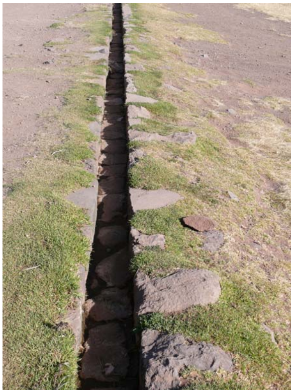
Fig. 9.26 The segment of restored channel bordering Inti-Huatana in Pisac (photo copyright by Yuri Gorokhovich). Color version available in Appendix
