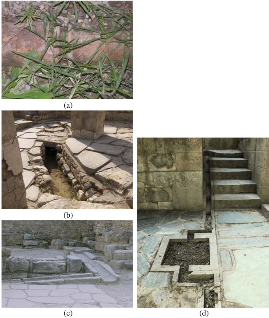
Fig. 1.5 Water components in Knossos. (a) Pipes made of terracotta. (b) Drainage channel. (c) Carved stone elements of rainfall harvesting system collecting water falling from roof. (d) Stepped water channel and sedimentation (desilting basin). Along the stairway is a small channel (for rain-water collection) consisting of a series parabolic-shaped stepped chutes that convey rainwater down stream to the sedimentation tank or basin (copyright permission with L.W. Mays). Color version available in Appendix
