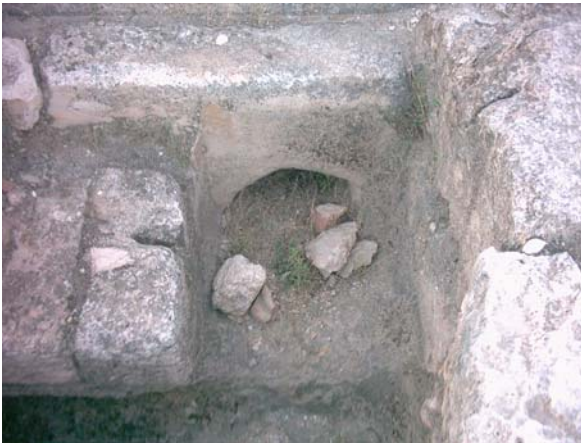
Fig. 8.10 Entrance of the water in the guard tower (point 2 in Fig. 8)
