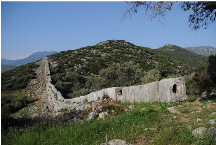
Fig. 1.10 Inverted siphon at Patara. Color version available in Appendix (copyright permission with L.M. Mays)
