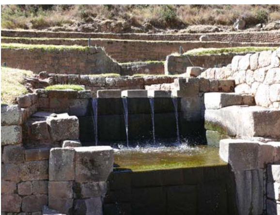
Fig. 9.20 Restored Inca fountain in Tipon. This is the principal fountain receiving water from the main spring in the background (photo copyright by Yuri Gorokhovich)
