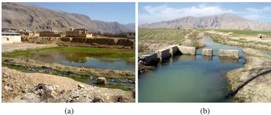
Fig. 5.3 (a) The outlet of Hasan-Abad subterranean canal is located in Seidan village (b) The earth conveyance canal of Hasan-Abad. Color version available in Appendix
