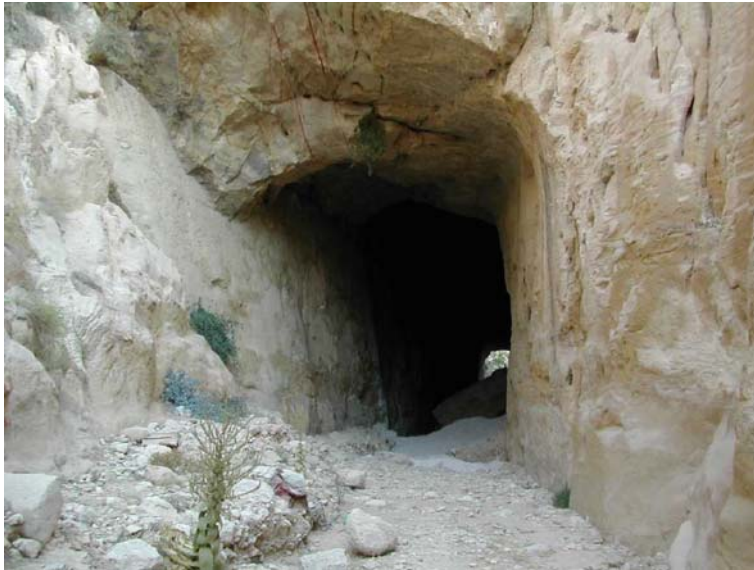
Fig. 1.17 Tunnel excavated by Nabataeans to divert flood water at the entrance of the Siq from Wadi Musa into Siq Mudhlim tunnel (photo courtesy of Mac McKee)
