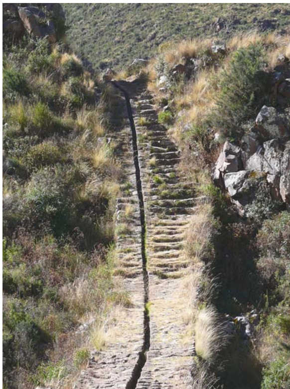
Fig. 9.17 Main aqueduct for Tipon. Note the stair steps on the steep terrain (photo copyright by Yuri Gorokhovich)
