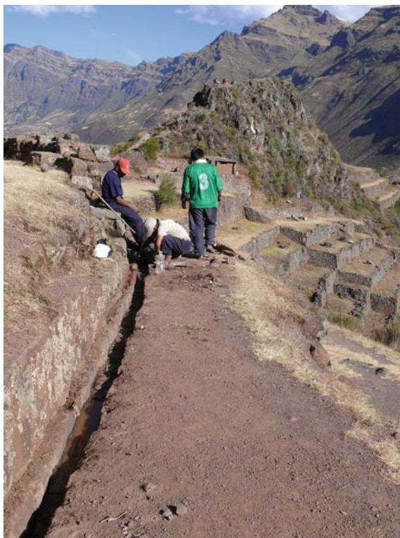
Fig. 9.27 Reconstruction of ancient water works often “masks” the original structure (photo copyright by Yuri Gorokhovich)
