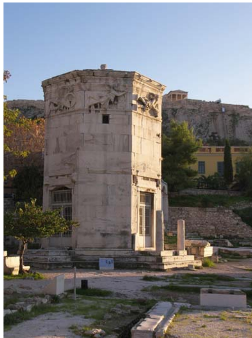
Fig. 1.13 Tower of the Winds. Located below the Acropolis in Athens, designed by the famous astronomer Andronikos of Kyrros to be an elaborate water clock (on the inside). The name is derived from the personifications of the eight winds carved on the eight sides of the building. Originally thought to have been built in the 1st century B.C. during the early Roman Empire, but now many archaeologists think the construction was in the mid-2nd century B.C. during the Hellenistic period (copyright permission with L.W. Mays)
