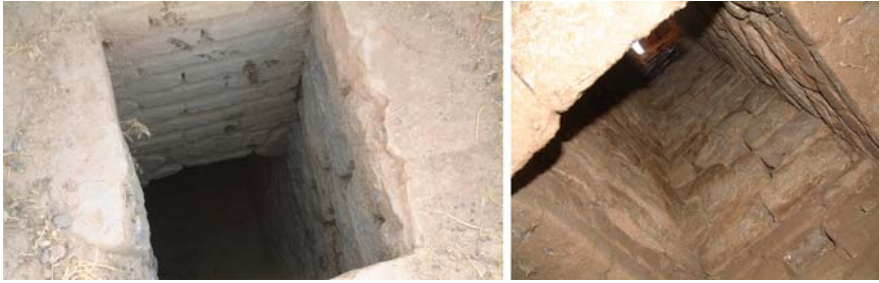
Fig. 5.5 Underground gutters at the northern platform
