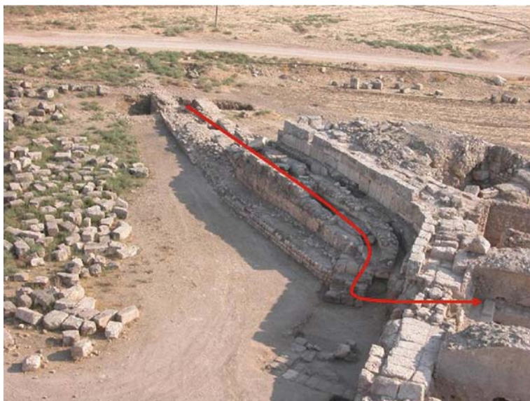
Fig. 8.6 Outer aqueduct delivering water into a cistern
