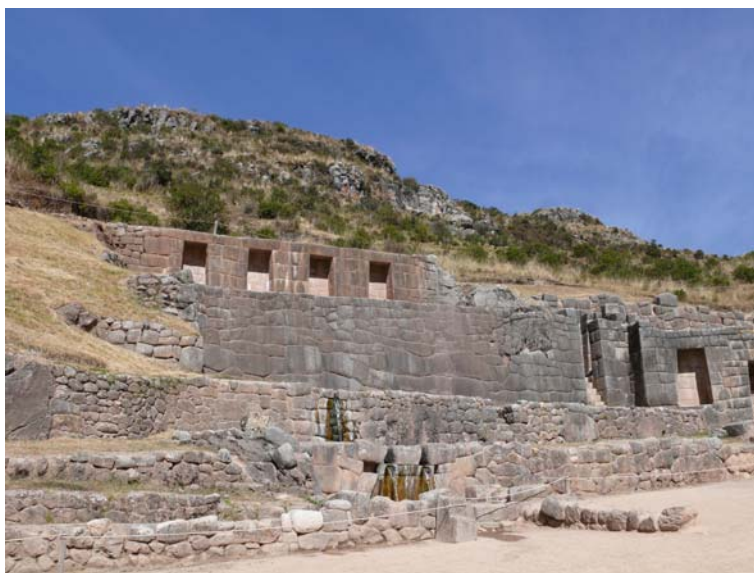
Fig. 9.28 Tambo Machay complex consisting of a retaining wall and a calvert with dual channels ( in the center of the picture ) (photo copyright by Yuri Gorokhovich). Color version available in Appendix
