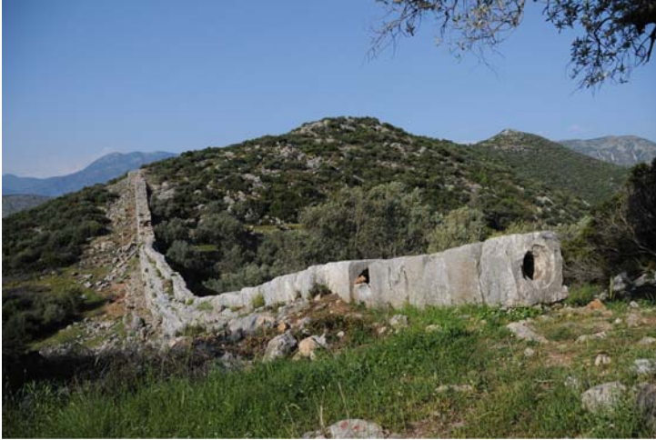
Fig. 1.10 Inverted siphon at Patara (copyright permission with L.W. Mays)
