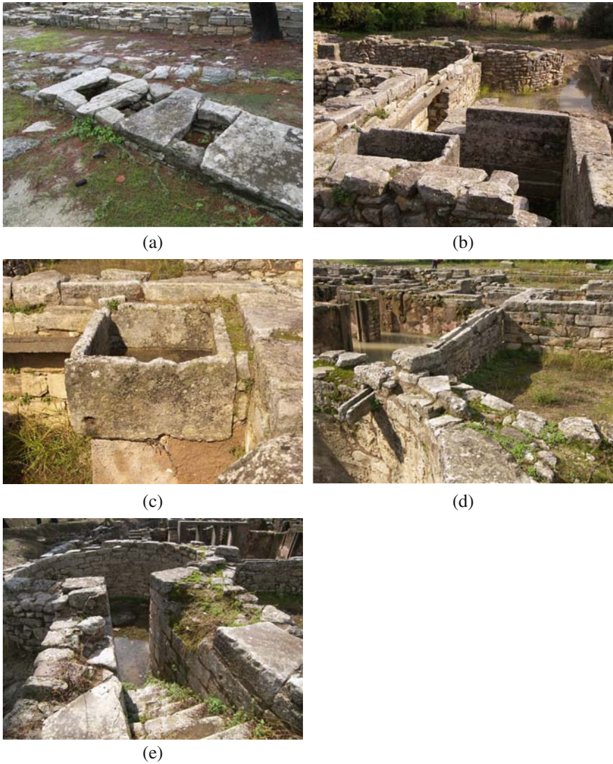
Fig. 1.7 Water system in Tyliisos, Crete. (a) Aqueduct bringing water from springs. (b) Sedimentation tank in foreground with stone channel connecting to cistern. (c) Sediment tank (d) Channel connecting sediment tank to cistern. (e) Steps leading down to cistern (photos copyright by L.W. Mays). Color version available in Appendix
