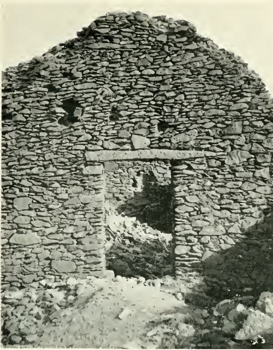
Mons Claudianus. Doorway leading from the hall of the Bath-house into the room in which was the plunge-bath. Originally the walls were plastered.—Page 125.
