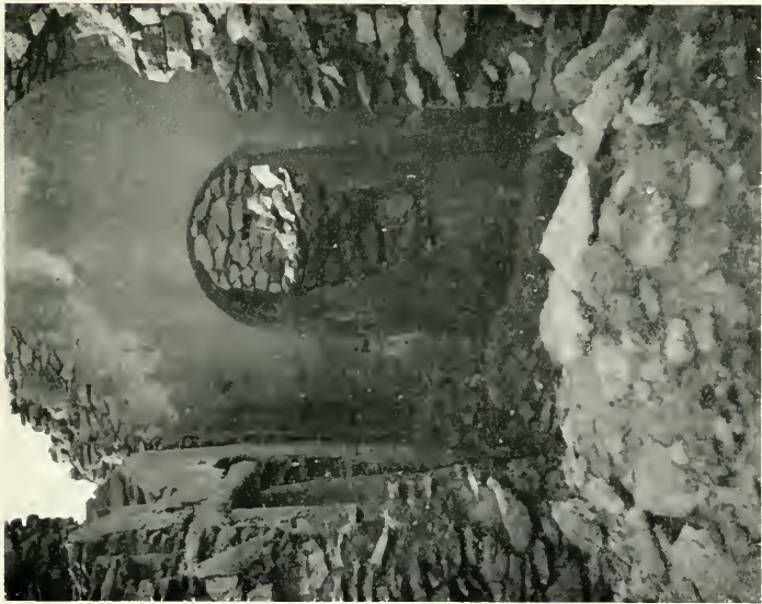
Mons Claudianus. The first heated room of the Bath-house. The doorway on the left leads into the warmer room. The perpendicular cut in the left wall near the corner is one of the recesses in which the hot-air pipes were fixed.—Page 125.
