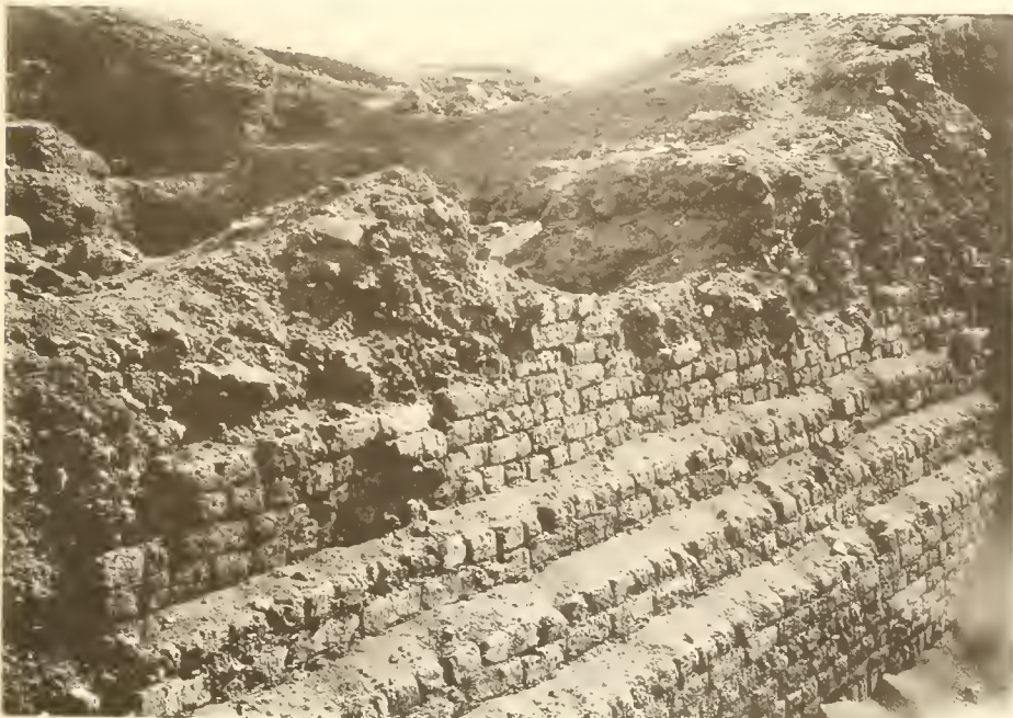
BLOCKING OF OLD ENTRANCE IN FOSSE.
