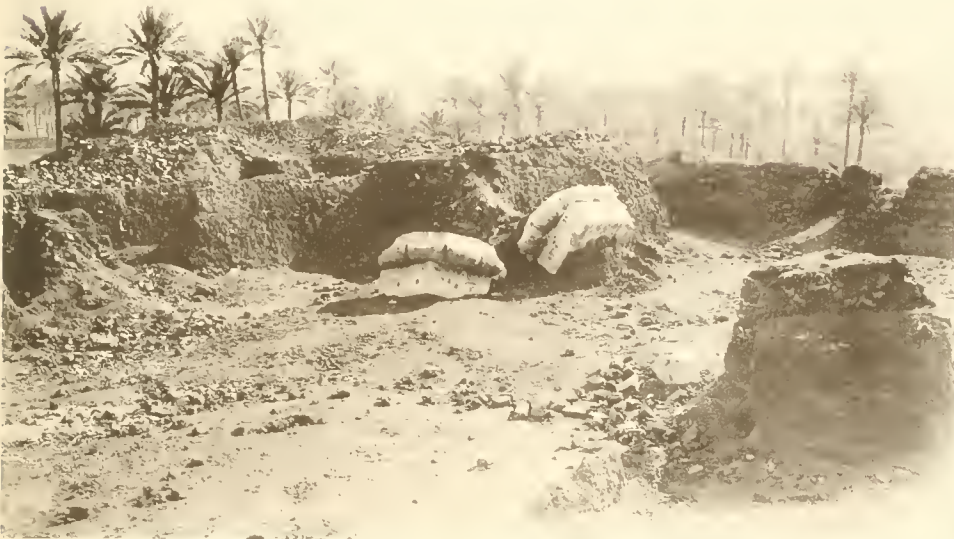
CAPITALS OF 50-FOOT COLUMNS, NORTH COURT.
