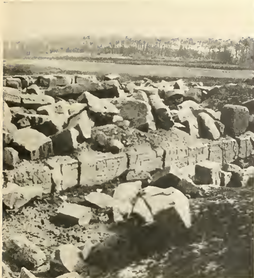
MAIN DOOR WAY.
