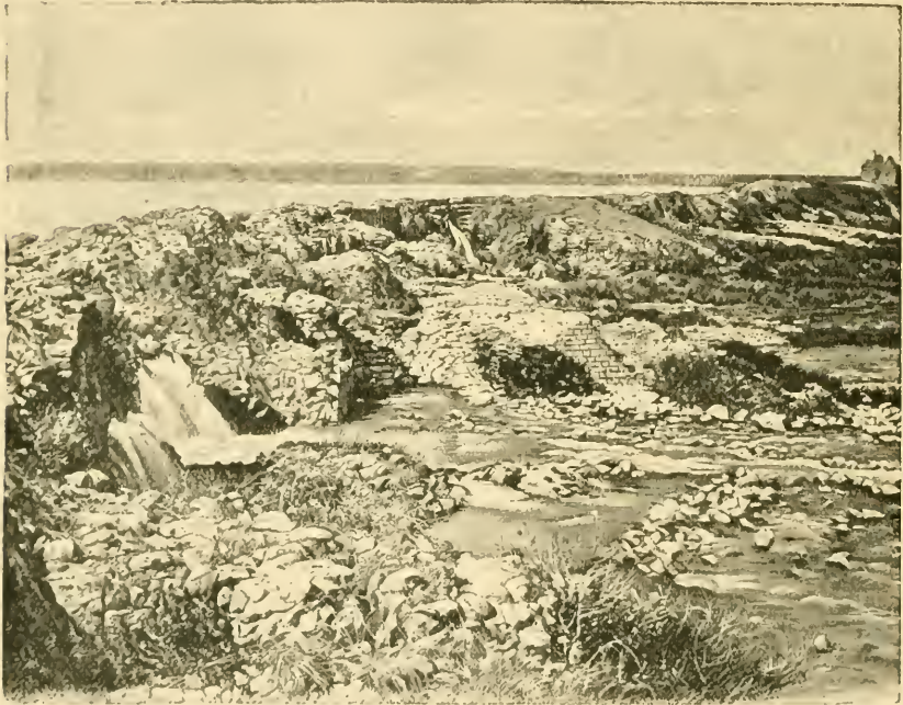
THE DYKE AT BAHR EL-KADES IN ITS PRESENT CONDITION. 1
