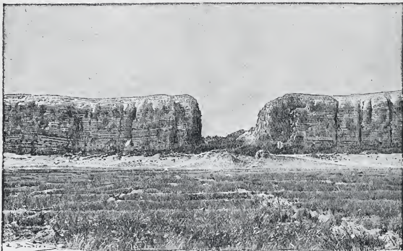
PART OF THE WALLS OF EL-KAB ON THE NORTHERN SIDE. 1
