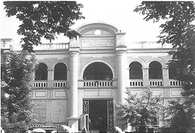
Plate 5.2 Main post office in Bamako, Mali. A fine example of French colonial architecture.
