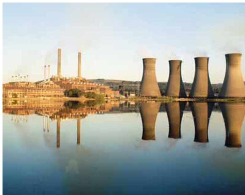
Energy production from coal is one of the largest contributors to CO 2 emissions. Power generation, South Africa.
