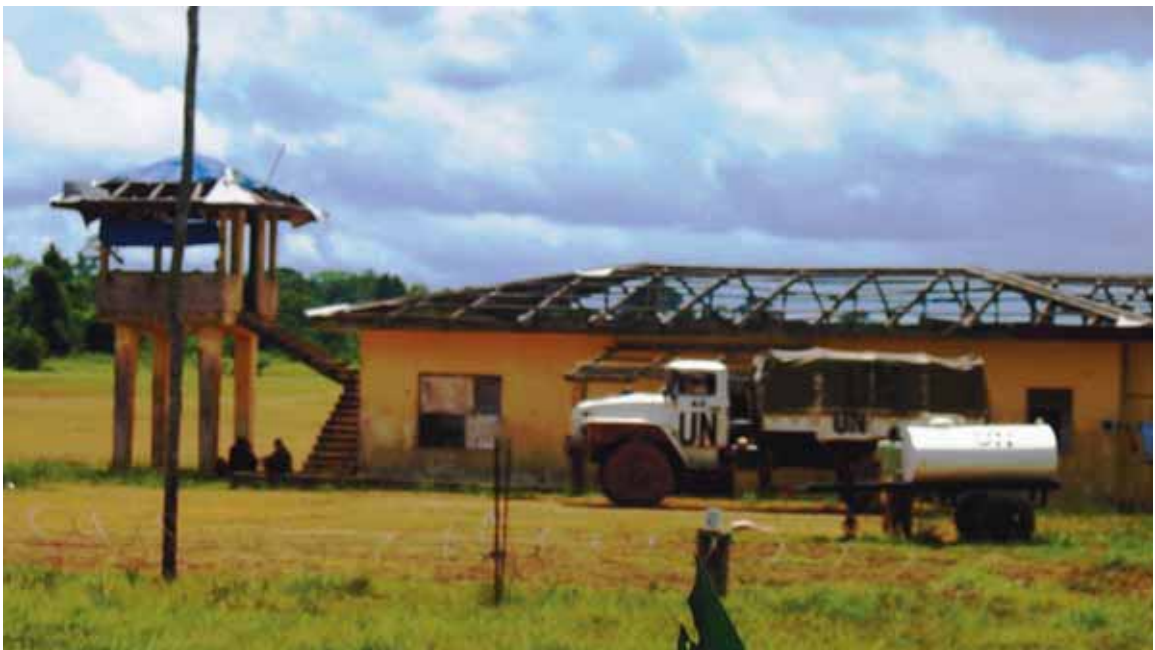
Infrastructural damage is a serious consequence of war and conflict. Shown here what remains of the airport at Greenville, Liberia, in 2005.
