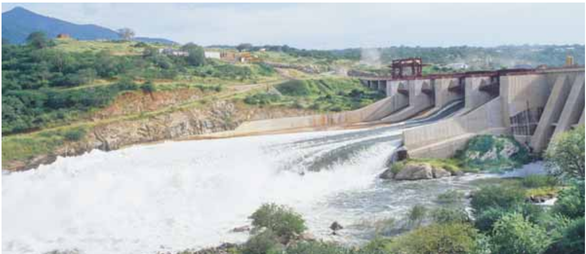
Hydroelectric dam, Tanzania.
