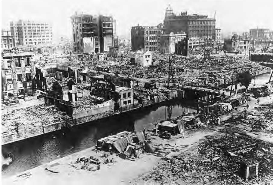
16. Little remained standing after the post-quake fires had raged for two days across Tokyo following the Great Kanto Earthquake of 1923
