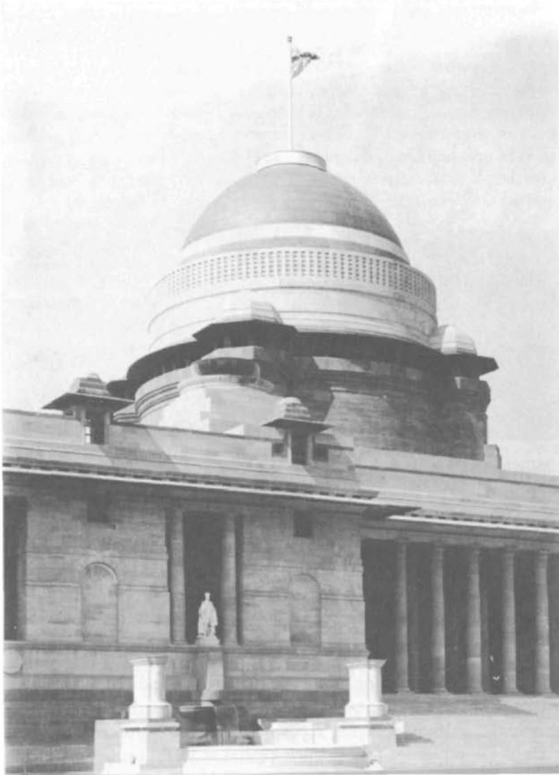
12 Viceroy's House, New Delhi (now Rashtrapati Bhavan), designed by Edwin Lutyens (1913–31). Note the use, together with the European-styled colonnade, of such Indic forms as the horizontal overhanging chajja, clustered chattris (cupolas), and a dome and encircling railing modelled on the ancient Buddhist stupa at Sanchi.
