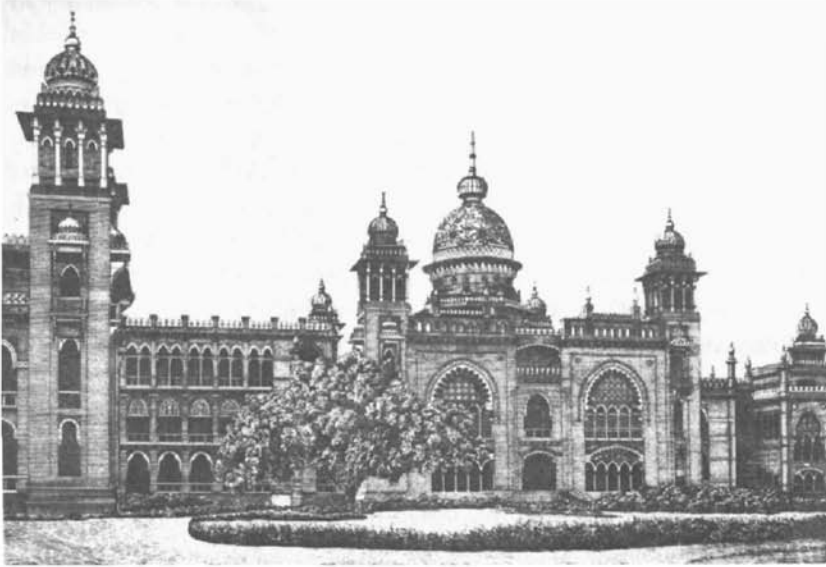
9 The Madras Law Courts , designed by J. W. Brassington and H. C. Irwin (1889–92). The structure, in the characteristic manner of the British Indo-Saracenic, joined together features, most notably arches and domes, from a variety of Indian styles, and incorporated as well arcaded verandas, colonnades, and a tower in the shape of a minaret containing a light to guide ships toward the nearby harbour. From Indian Engineering , 7 September 1895.
