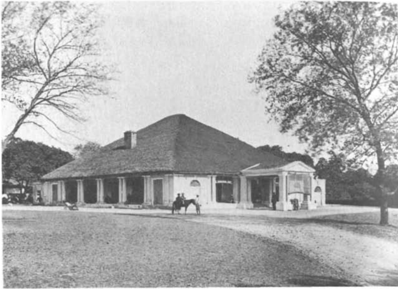
13 Bungalow, Allahabad (1866). Note the expansive thatched roof, encircling verandah, and placement in the centre of a large compound with curving entry way.
