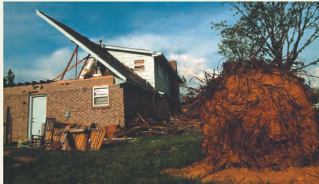
F1: 33–50 m/s (73–112 mph); surface of roofs peeled away; windows broken; trees on soft ground uprooted; trailer houses moved or overturned
