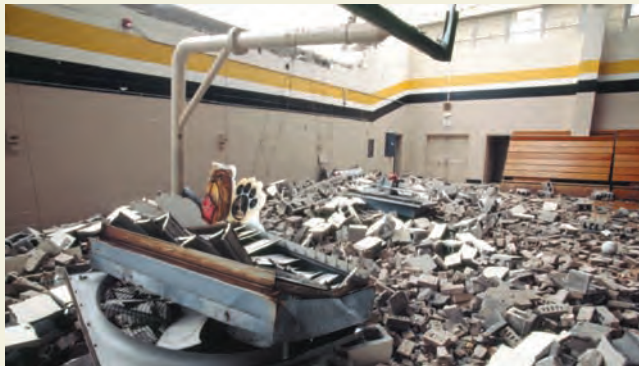
F3: 71–92 m/s (158–206 mph); roofs torn off well-constructed houses; some rural buildings completely demolished; steel-framed, warehouse-type structures badly damaged; cars lifted off the ground; most trees uprooted or leveled
