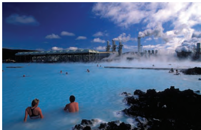
12.18 Geothermal power plant
