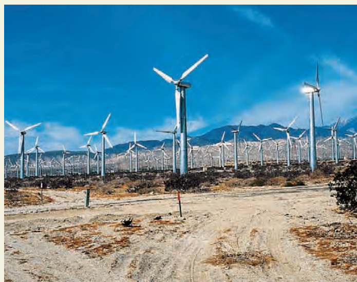
▲ Modern windmills A wind farm in San Geronio Pass, near Palm Springs, California. Wind speeds here average 7.5 m/s (17 mi/hr). Wind farms use wind turbines with a generating capacity in the range of 50 to 100 kilowatts.
