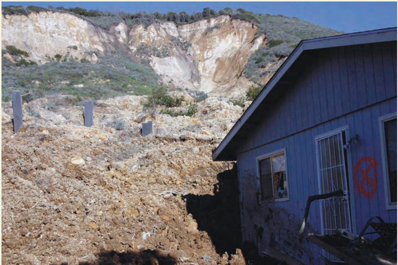
▲ Earthflow at La Conchita Nestled between the beach and a high bluff of unstable regolith, the town of La Conchita, California, has experienced periodic earthflows following heavy rains for several decades. The most recent earthflow, in 2005, overtopped a fortified retaining wall, marked here by the three steel I-beams projecting above the ground. The earthflow pushed this home off its foundations.
