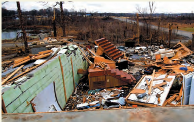
F4: 93–116 m/s (207–260 mph); well-constructed houses leveled, leaving piles of debris; structures with weak foundations lifted and blown away; cars blown large distances; large projectiles generated
