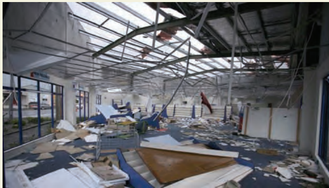
F2: 51–70 m/s (113–157 mph); roofs torn off frame houses; weak structures or outbuildings demolished; large trees snapped or uprooted; cars blown off highways; walls badly damaged but standing
