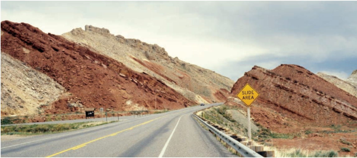
■ FIGURE 12.32 Rock units that dip in the same direction as the topographic slope of the land are especially susceptible to rockslide, as recognized along this stretch of highway in Wyoming.
