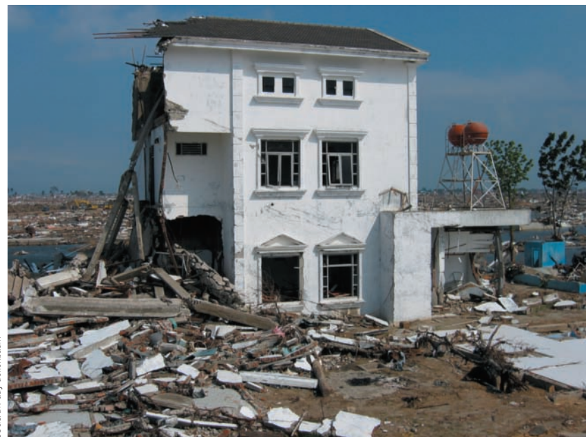
■ FIGURE 11.34 The 9.1 magnitude Sumatra–Andaman earthquake, and the tsunami that it generated, devastated the city of Banda Aceh on the Indonesian island of Sumatra. Here, above the lowest set of windows, the only piece of a building left standing displays dark scratches made by debris carried in the tsunami.
